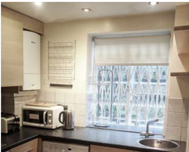
Fig. 18 Existing window removed wall knocked through under cill and completely to right-hand-side of window. Vestigial wall nib to left-hand-side partially retained (LG05)
