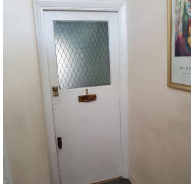
Fig. 21 Existing front door to flat to be replaced (Hall UG01)
