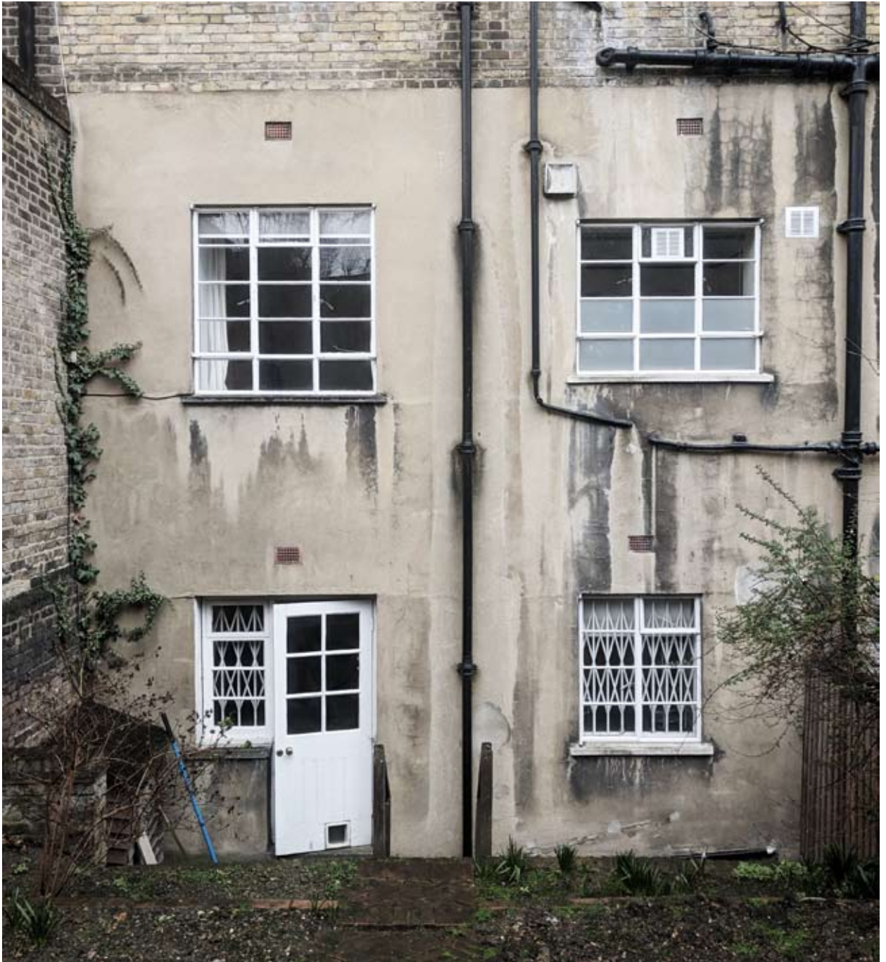
Fig. 24 Rear-elevation - Existing render patch repaired to match existing finish.
