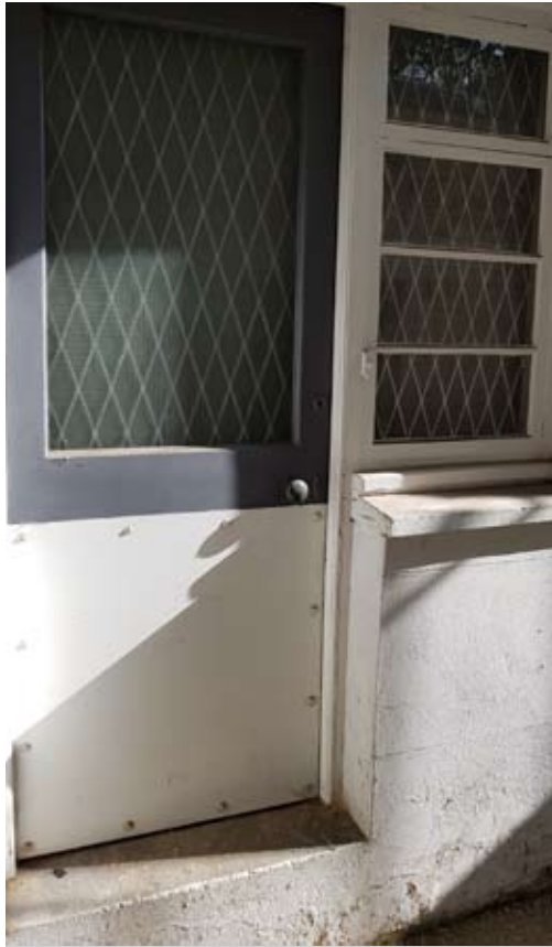
Fig. 11 Existing front door and sidelight window to be replaced (external view)
