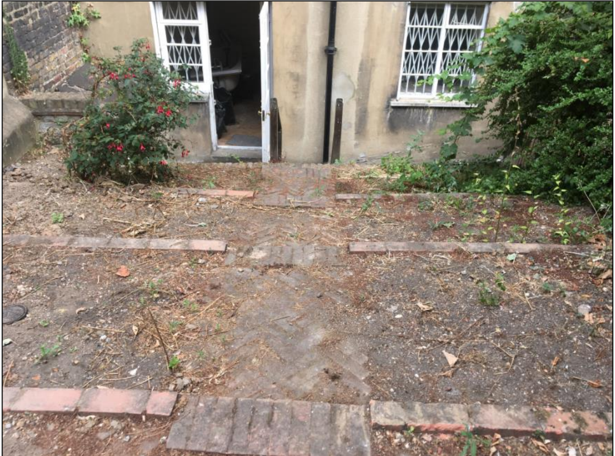
Photo 1: Existing stepped back garden of property. Note the garden is mainly hardstanding.
