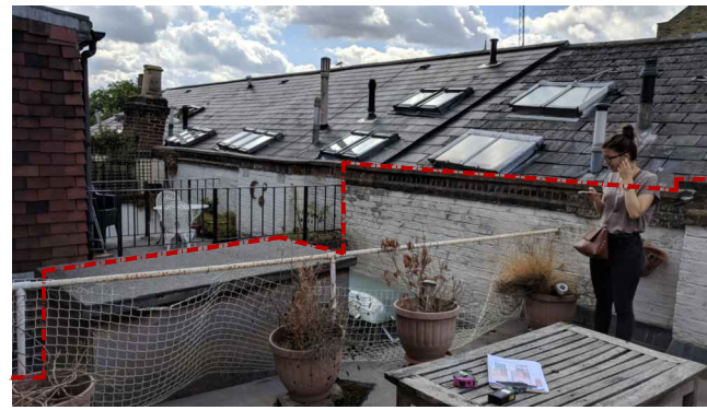
Existing roof terrace at 81 Haverstock Hill
