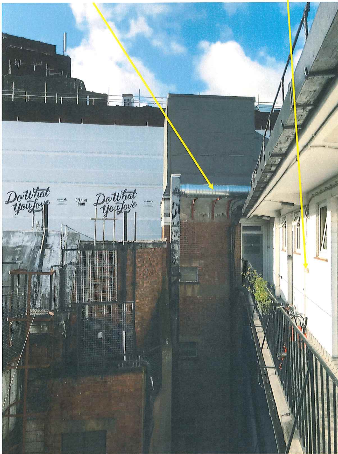
Photo D – Top of lightwell behind residential flats at Phoenix House
