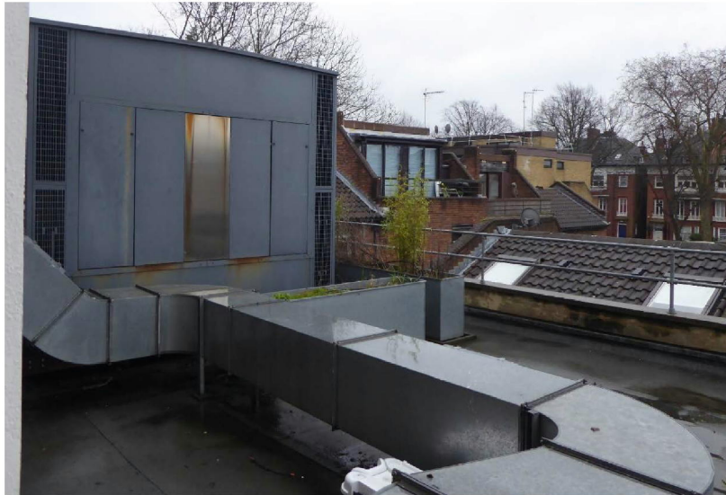
The plant comprises an extraction duct in relation to the restaurant, as well as extraction/ventilation equipment enclosed with housing and screened with planters.
