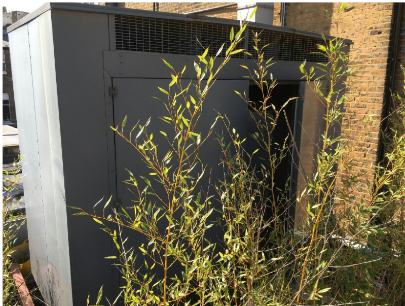
The plant comprises an extraction duct in relation to the restaurant, as well as extraction/ventilation equipment enclosed with housing and screened with planters.
