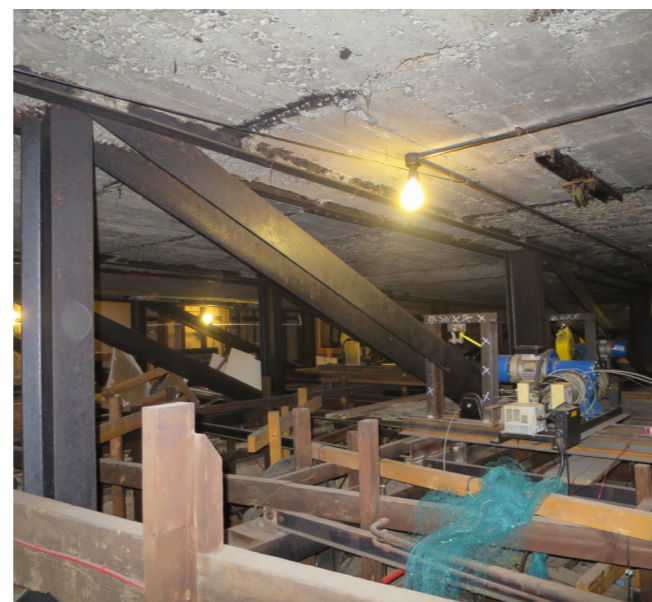
Existing roof structure over KOKO auditorium
