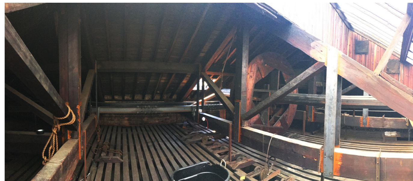
Photo of existing flytower roof structure
