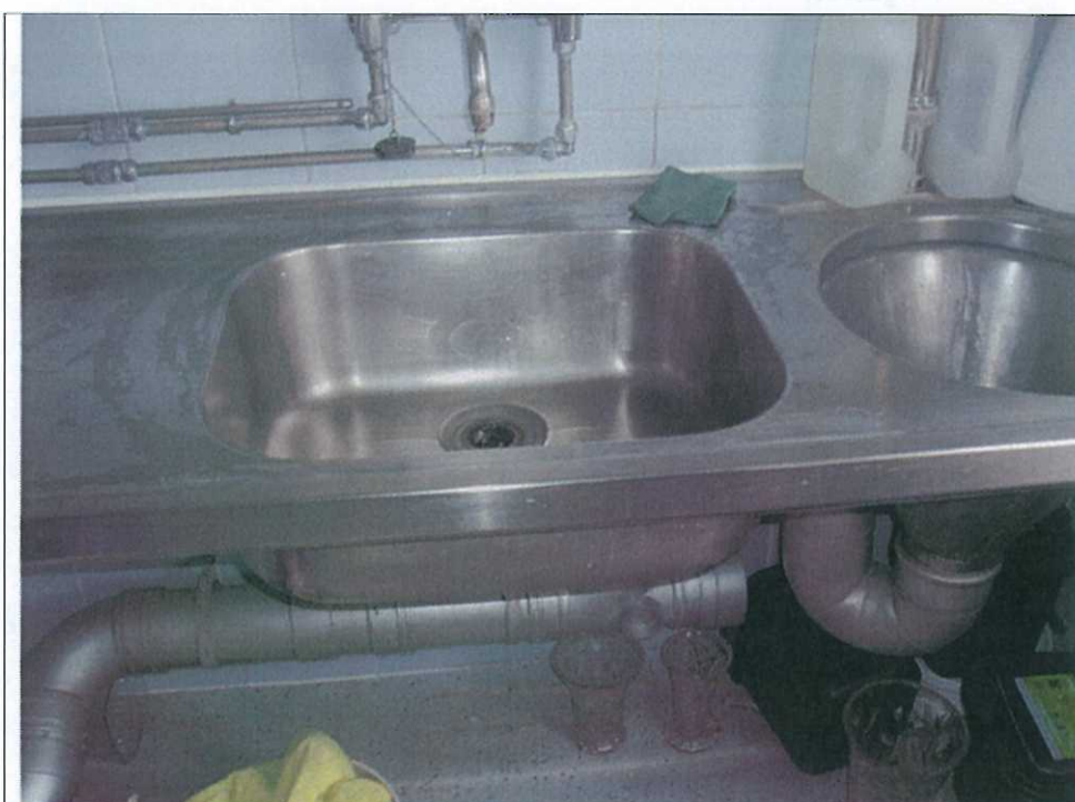
MER00590/I.R/06. Ground floor, sluice room and cleaners cupboard. Rumble pads to sinks.
