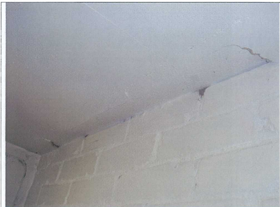
MER00590/I.R/11. Lift motor room. A.I.B. infill to ceiling.
