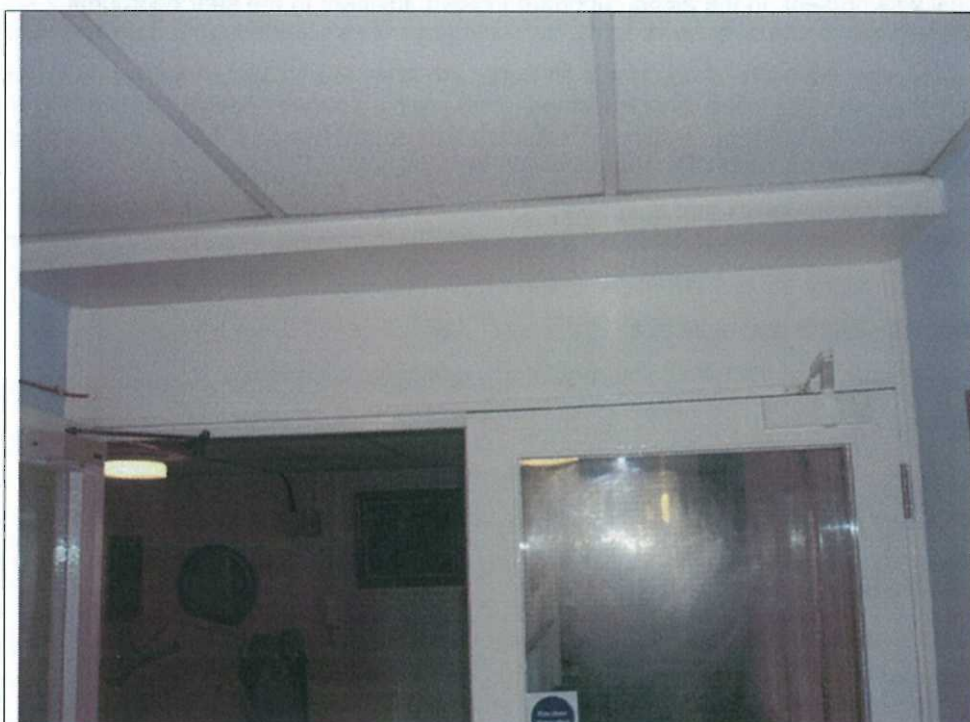
MER00590/I.R/02. Lower ground floor. Insulation board infill panel above doors within main corridor.
