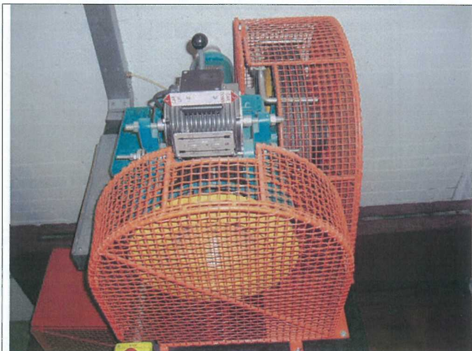
MER00590/I.R/10. Lift motor room, brake shoes to lift motor.
