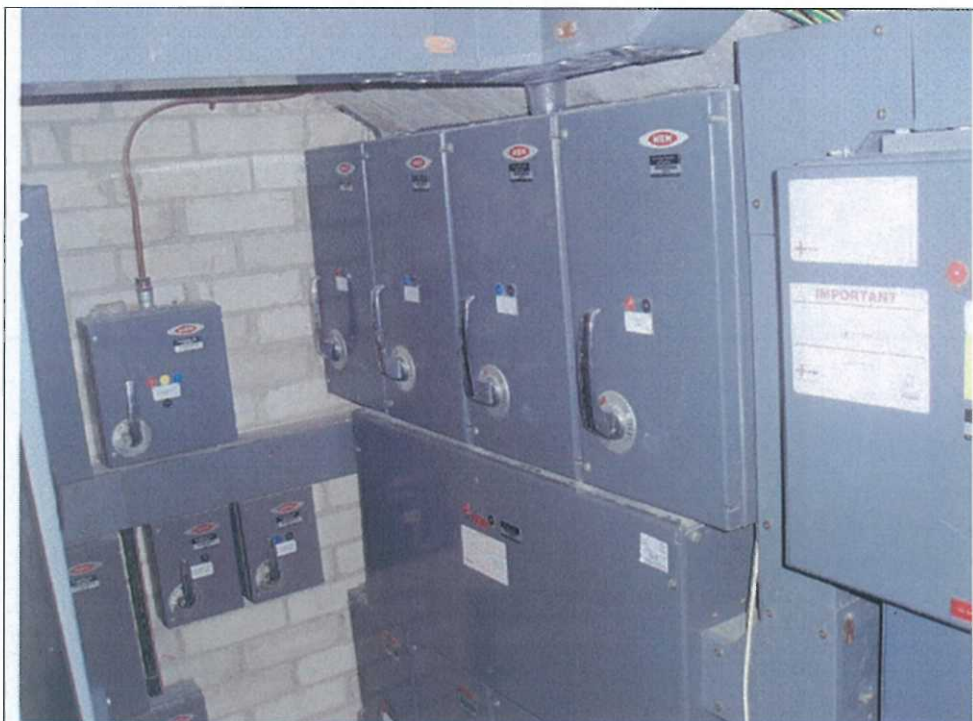
MER00590/I.R/03. Electrical intake room, fuse boxes with possible asbestos flash guards.
