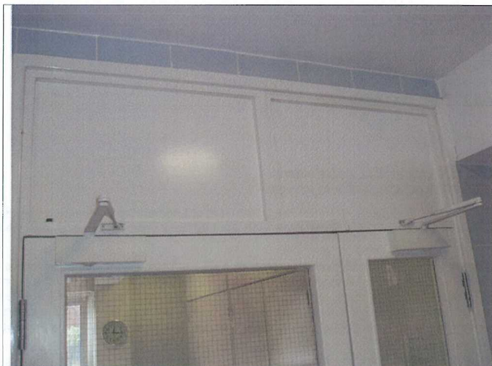
MER00590/I.R/01. Lower ground floor. Insulation board infill panels above doors to laundry area.
