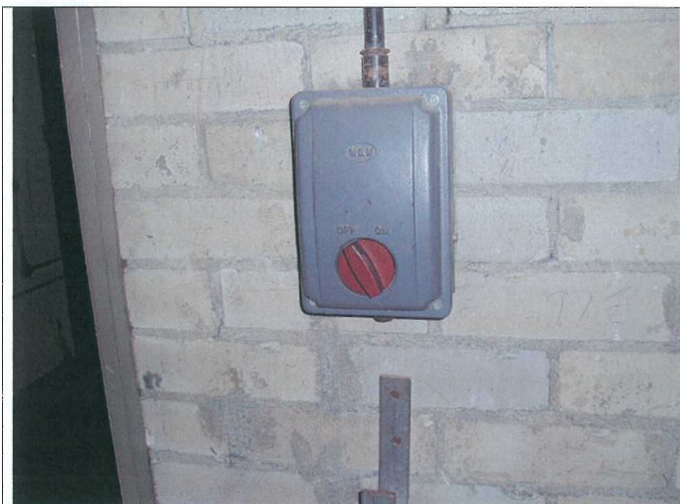
MER00590/I.R/12. Tank room, fuse boxes that may contain asbestos.
