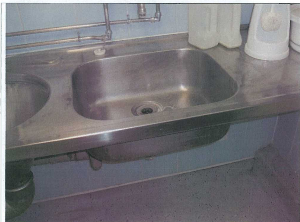
MER00590/I.R/04. Lower ground floor, sluice room. Sinks with bitumen rumble pads attached.
