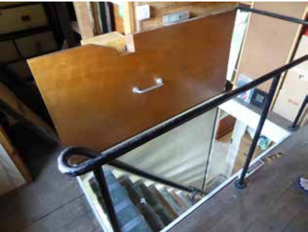
LANDING HATCH TO BE REMOVED AND NEW STUD WALL ERECTED TO FOR NEW BATHROOM AND BOILER
