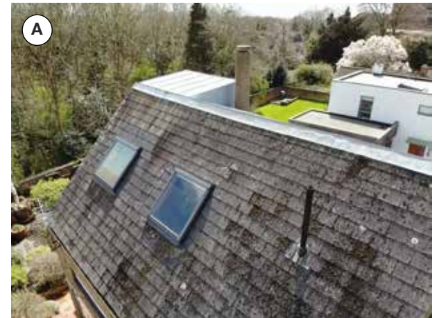
ASBESTOS ROOF TILES TO BE REMOVED AND NEW TILES INSTALLED TO MATCH EXISTING (IN APPEARANCE)
