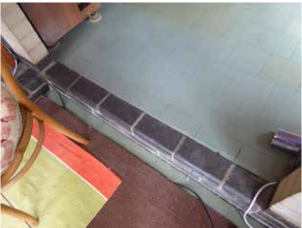
NEW WOOD FLOORING TO PLAY ROOM - BRICK THRESHOLD TO BE MAINTAINED
