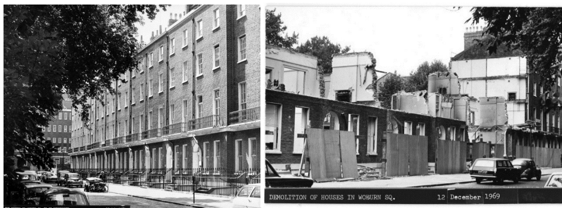
Fig. 4 & 5 – Woburn Square Georgian terraces to be demolished (1969), Woburn Square terraces being demolished to make way for the Philips Building (1969) [SOAS Picture Archive 2018]
