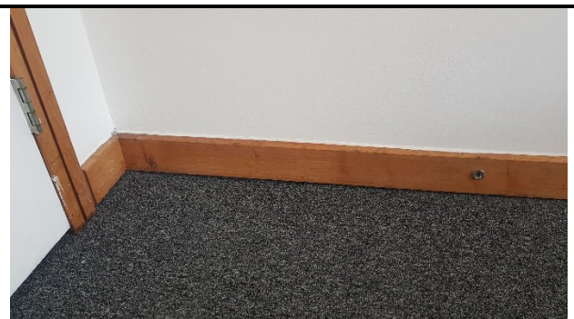
Fig. 12 – Existing finishes to academic office floors
