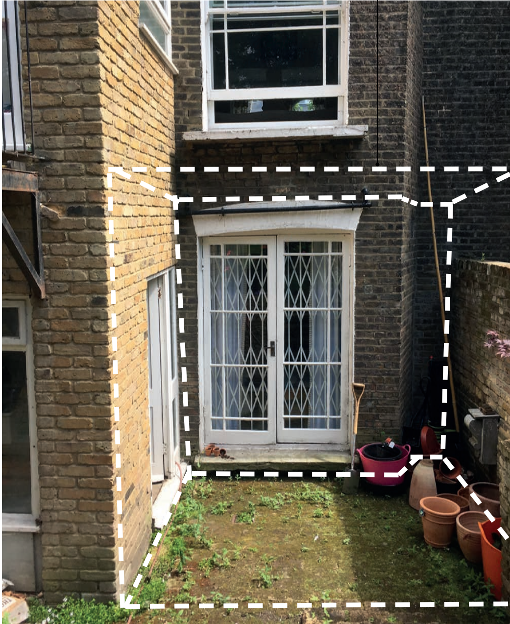
View of 81 St Augustine's Road lower ground floor garden elevation. Full width extension outlined.
