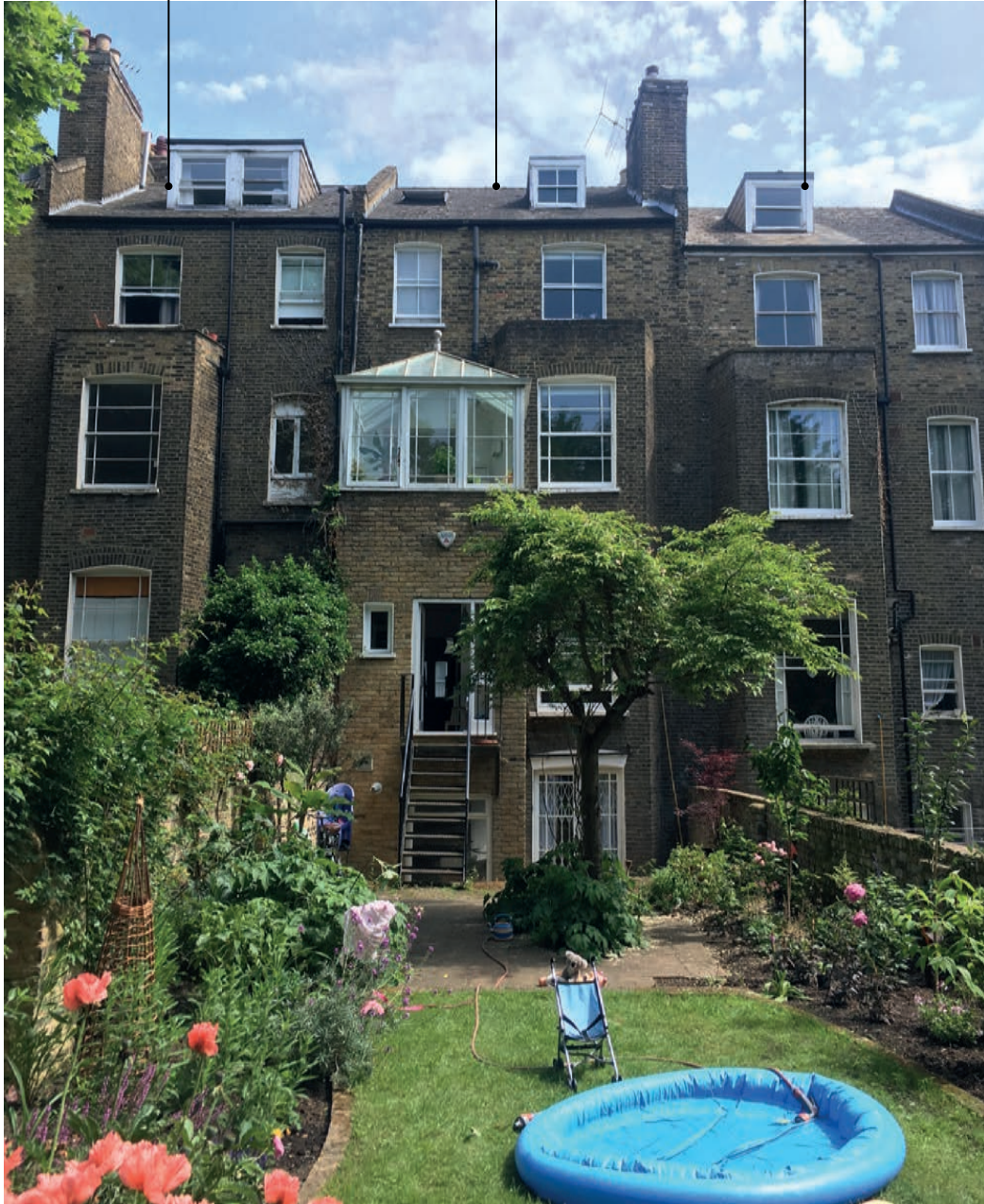
View of 81 St Augustine's Road rear elevation.
