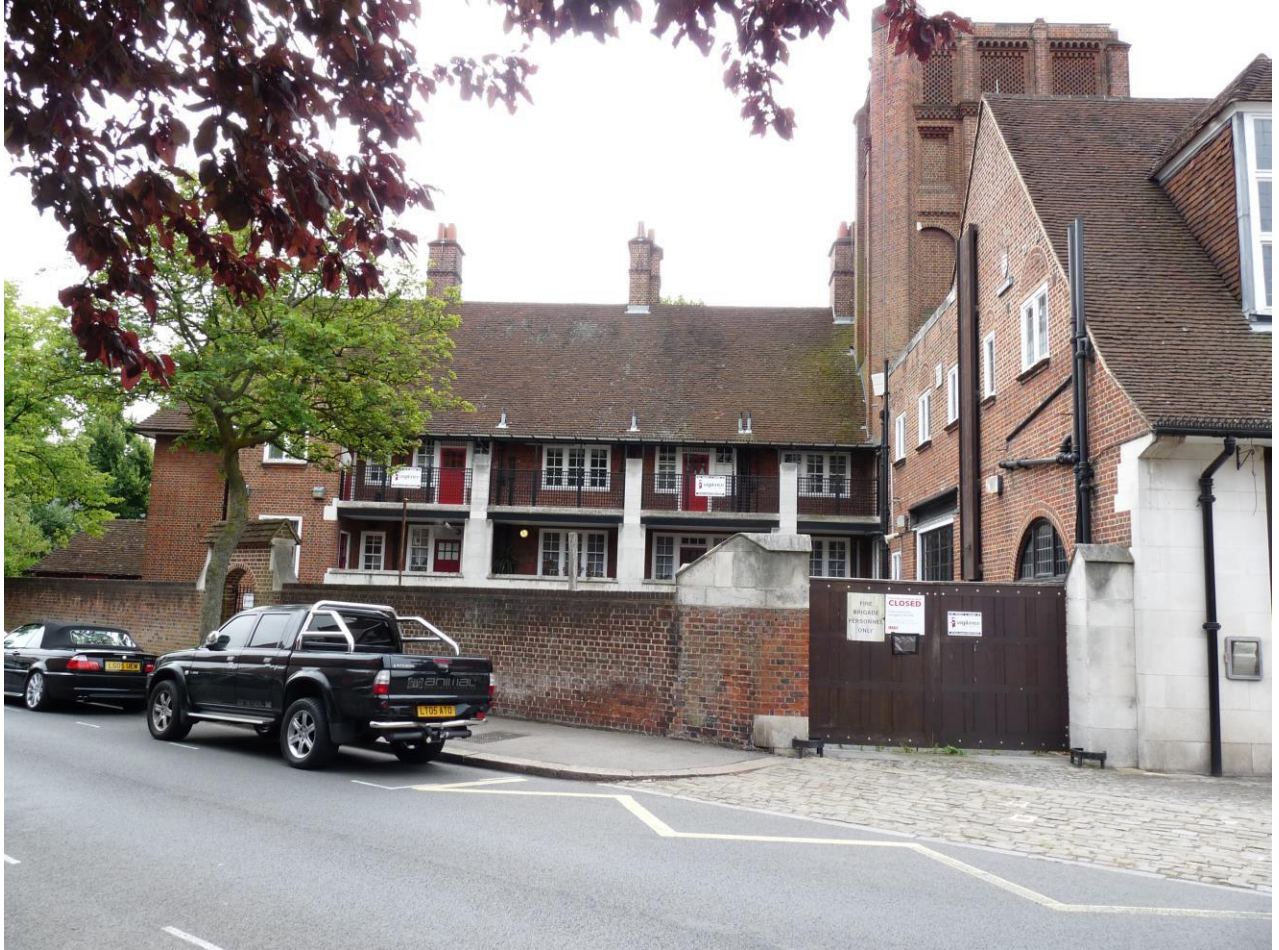
Fire station viewed from Lancaster Grove
