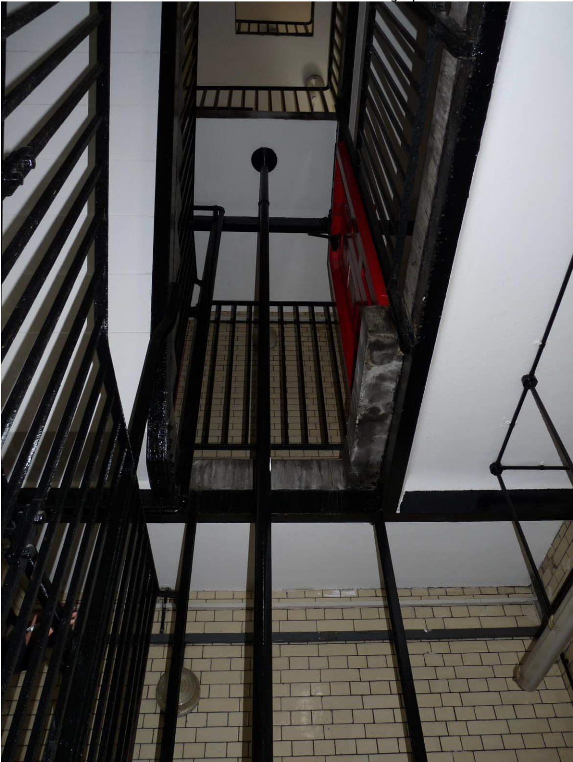
Photograph of stair tower interior
