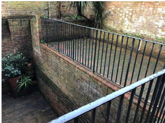
Rear Garden - ground floor terrace with view of basement level terrace
