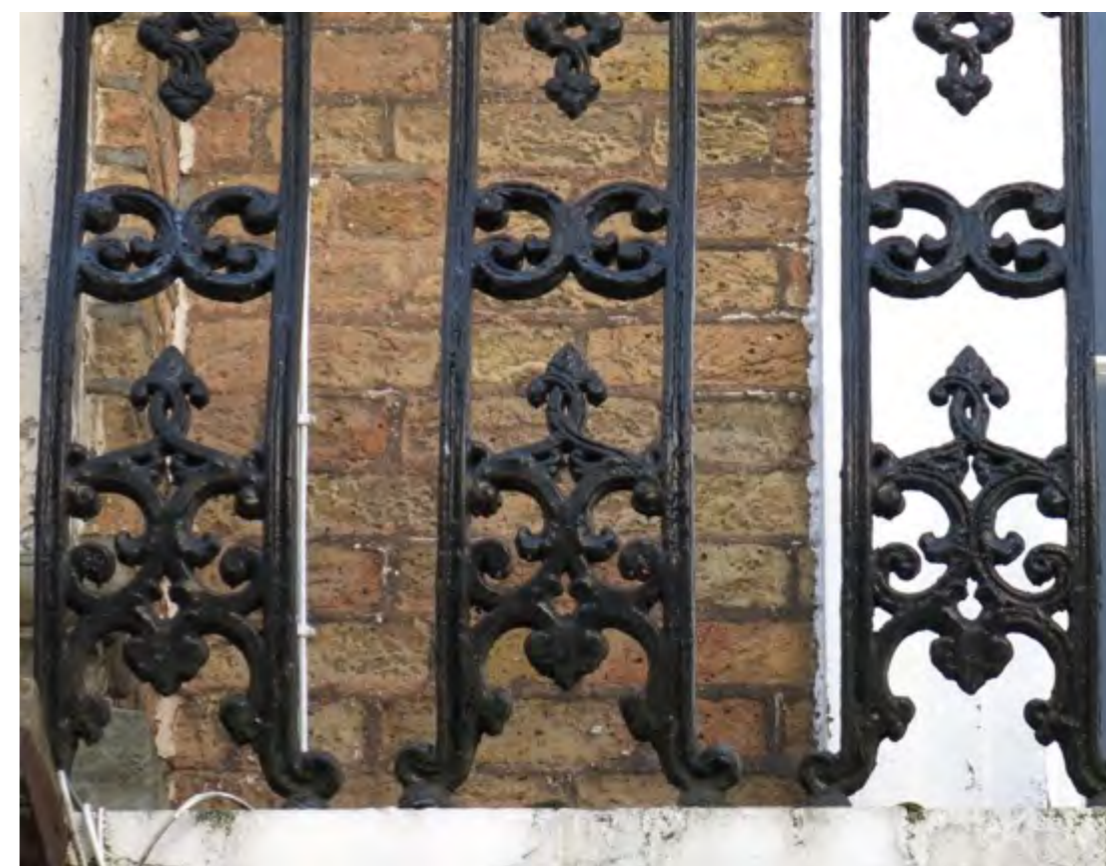
Figure 5. Original coloured flush mortar joints with remnants of white 'Tuck pointing' at 32 Mornington Terrace
