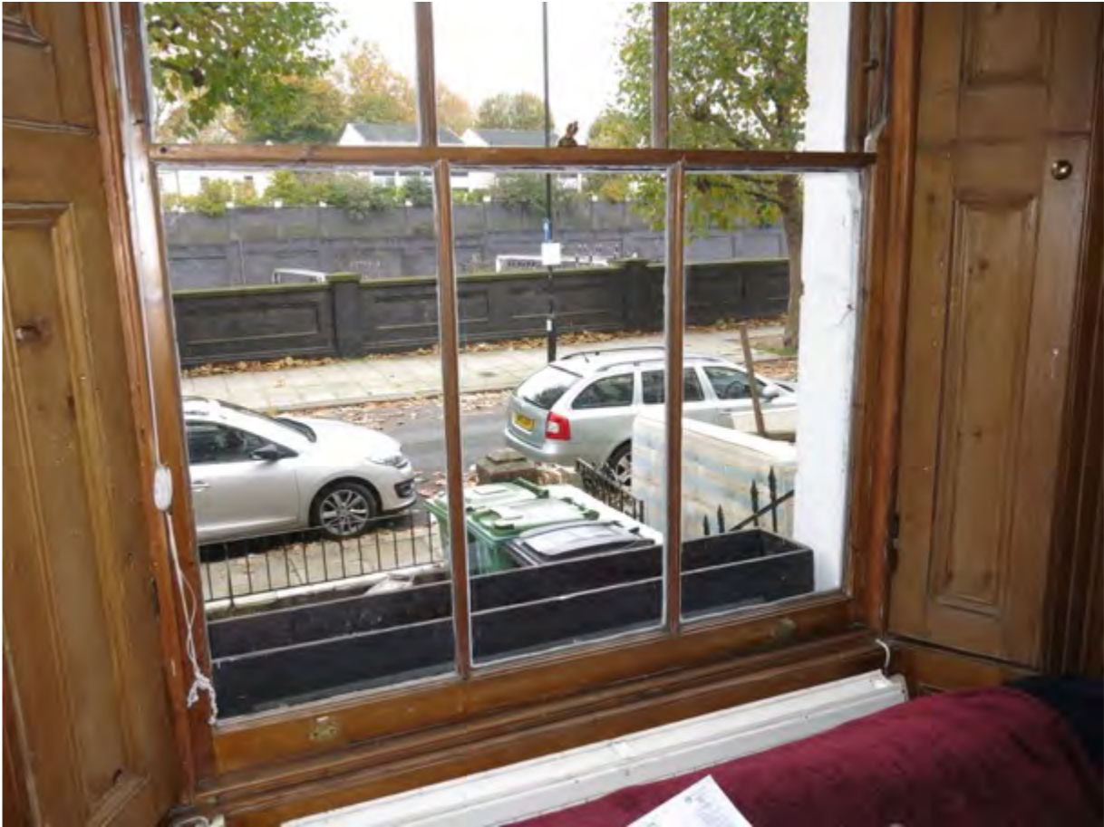
Figure 13: View of the bottom sash and internal window cill
