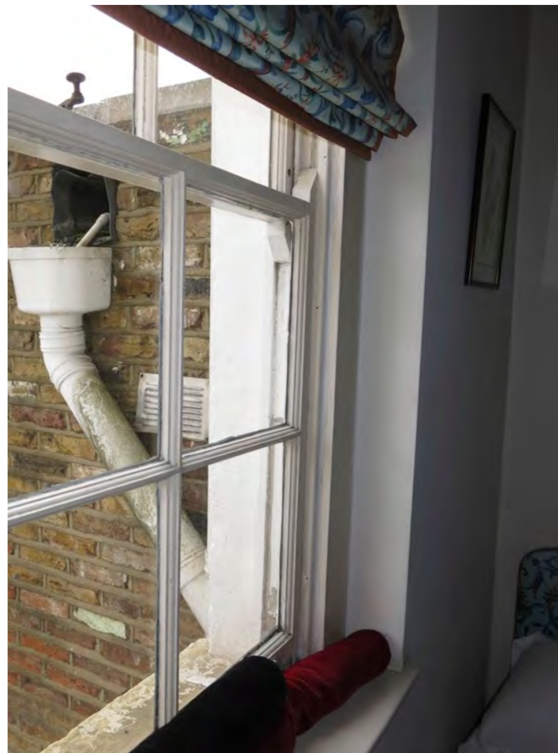
Figure 15: The internal plastered window reveals
