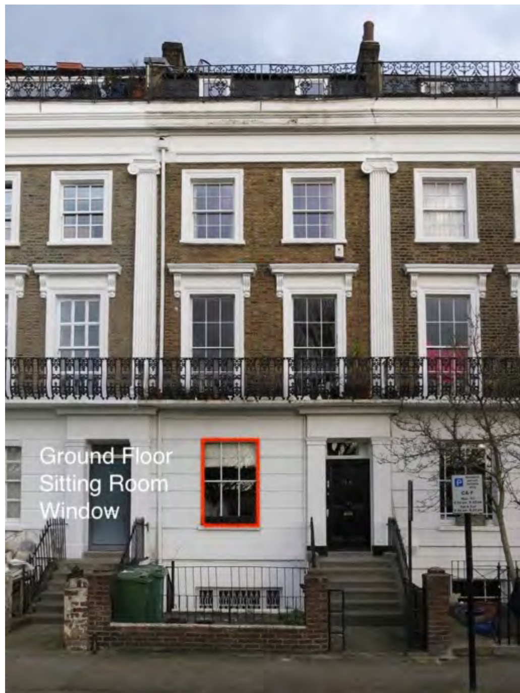
Figure 8: A view of the front elevation of 28 Mornington Terrace. Windows where internal secondary glazing will be installed are annotated in RED . The rear elevation was not accessible to take an external photograph.
