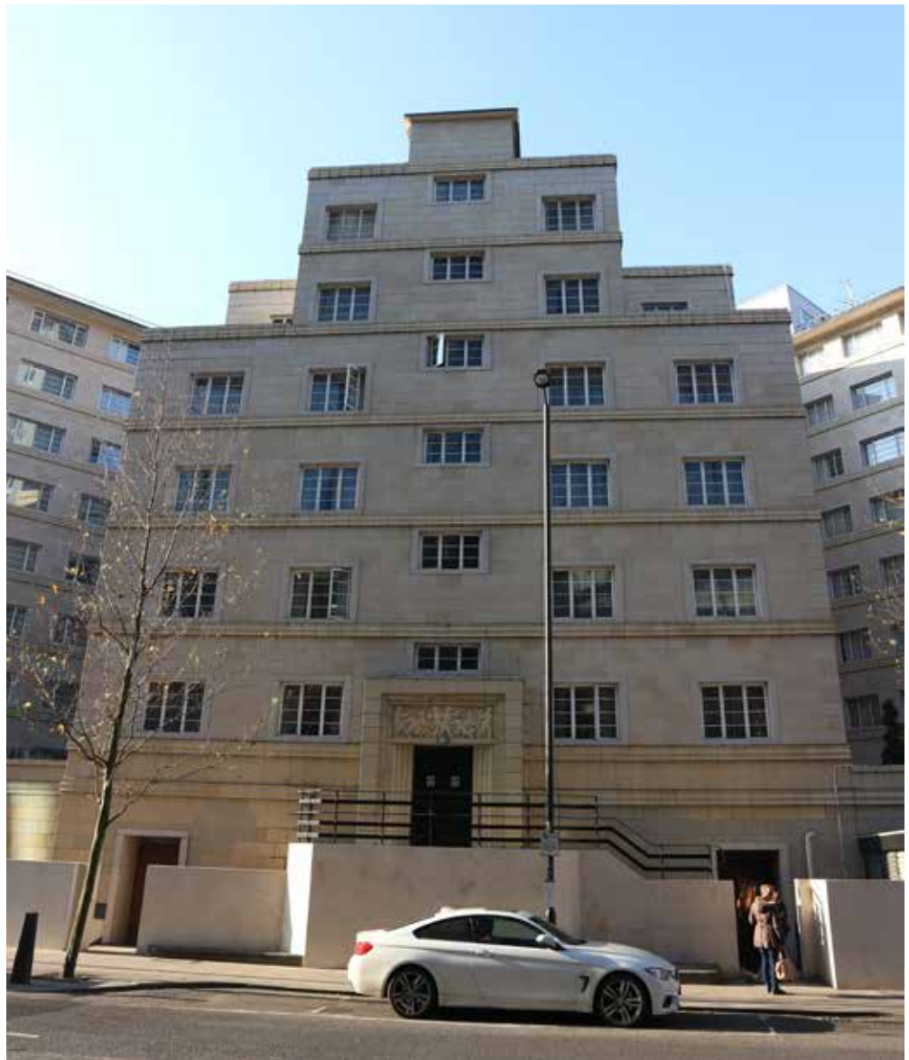
22. End Elevation, Central East Wing (Insall, 2017)
