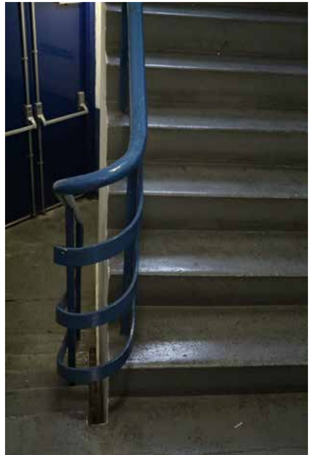
24. Service Staircase, South-West Wing (Insall, 2018)
