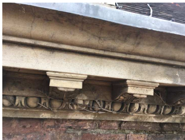
Figure 5: Heath House, Existing Eaves Cornice
