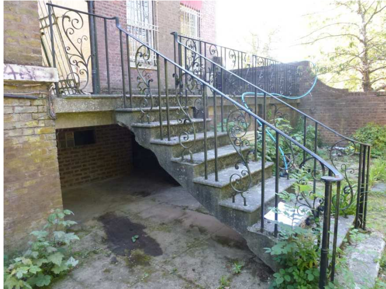
Figure 4: Existing terrace, stair and railings
