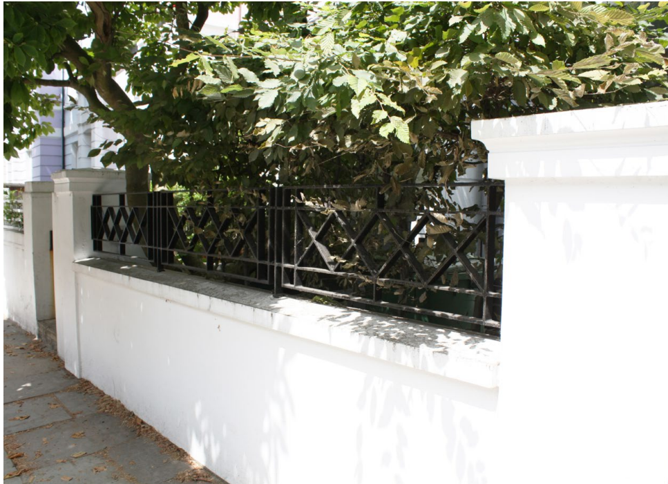
Fig. 17: The rendered boundary wall with metal railings and planter to 12 Regent's Park Road
