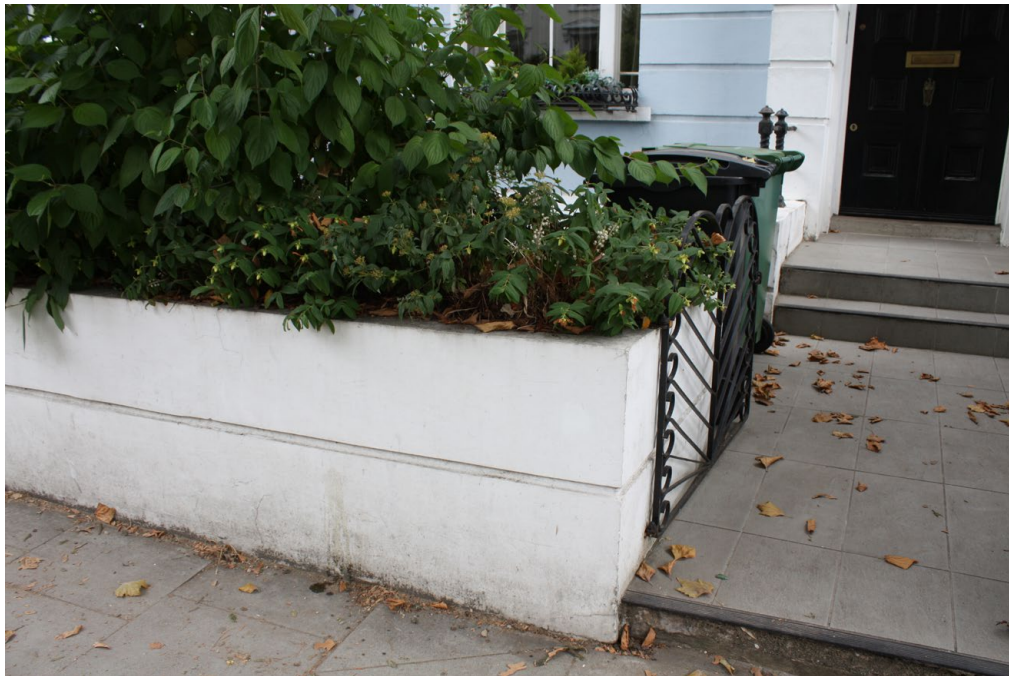
Fig. 10: The ground floor entrance, with the current bin store partially visible
