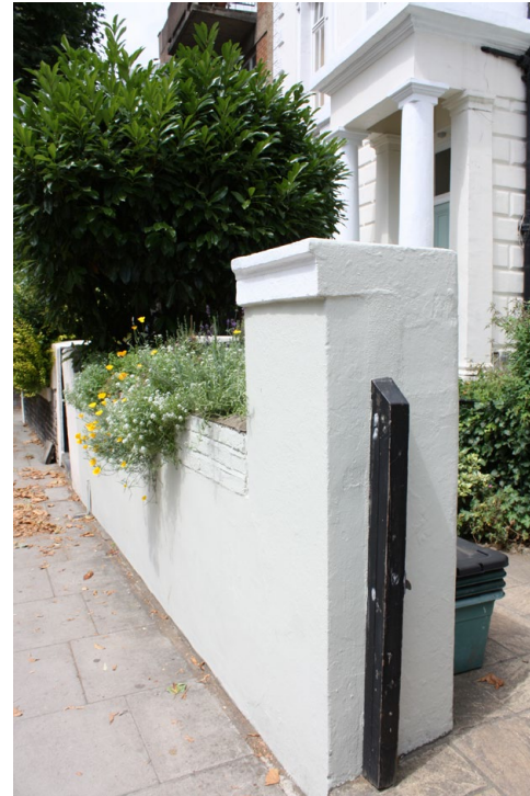
Fig. 20: The rendered boundary wall to 6 Regent's Park Road, featuring planters to the street scene
