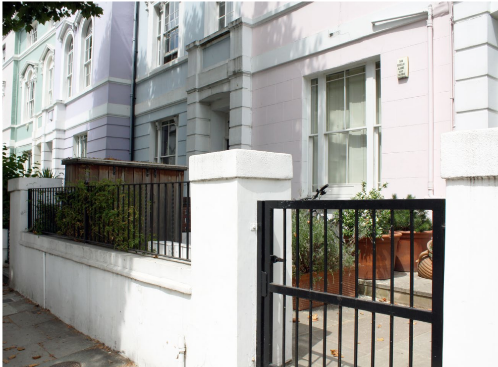
Fig. 14: 14 Regent's Park Road, featuring a rendered boundary wall with metal railings and vegetation, and rendered piers to the entrance gate
