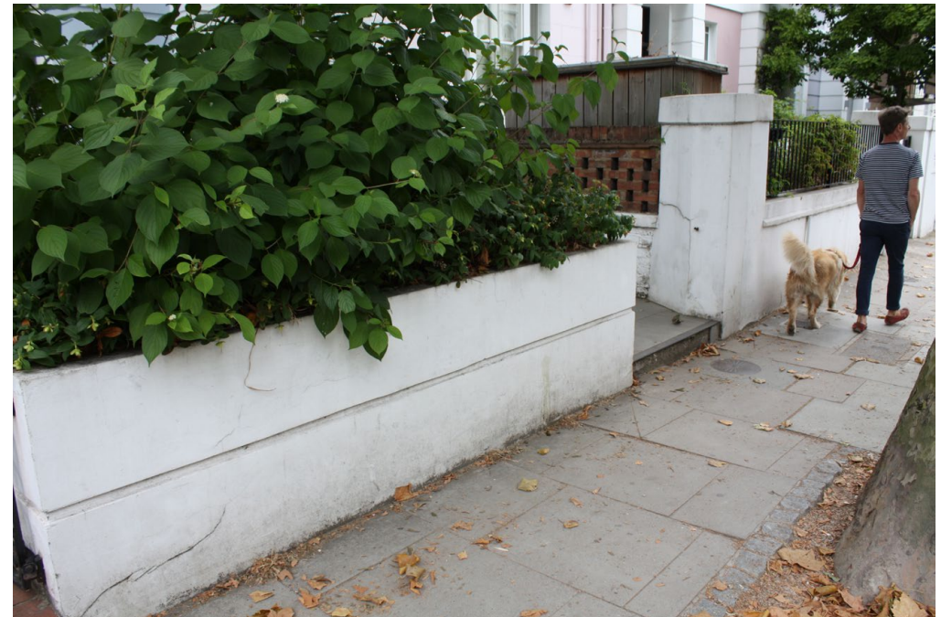
Fig. 09: The existing street elevation, showing the boundary wall with planter behind
