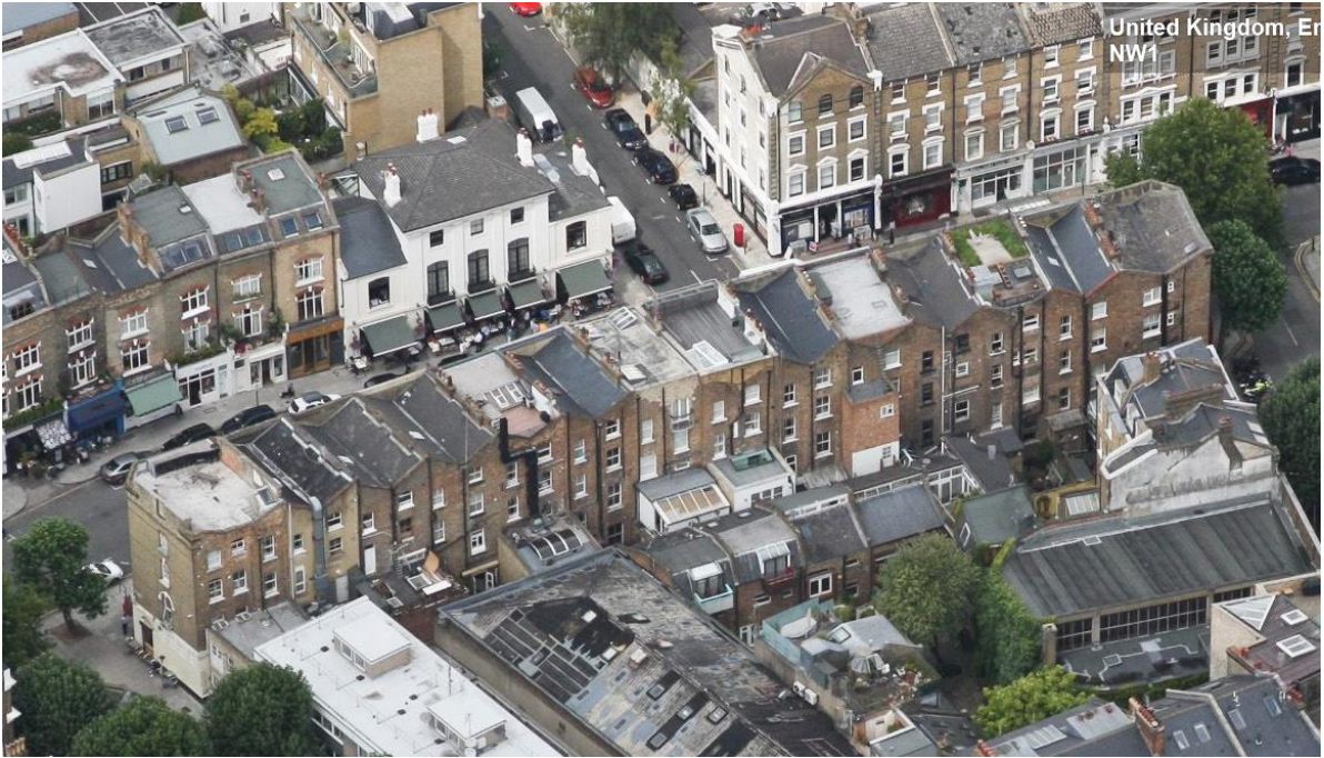
Figure 1: Nos. 146 to 172 (even) Regent's Park Road showing a clear pattern of low scale rear extensions within the terrace, with the exception of No. 164 (centre right).
