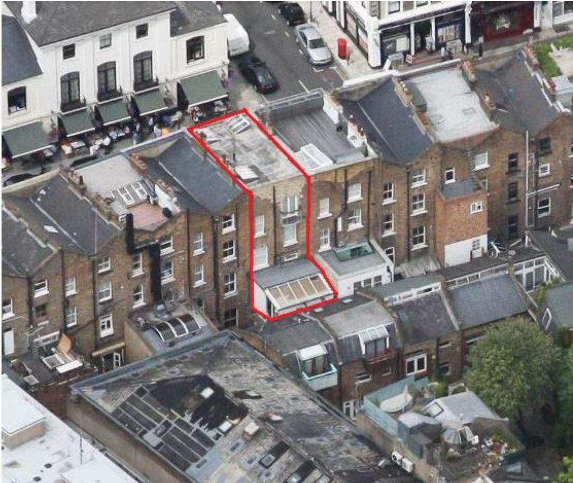
Figure 2: 158 Regent's Park Road in rear view with first to third floors outlined in red.
