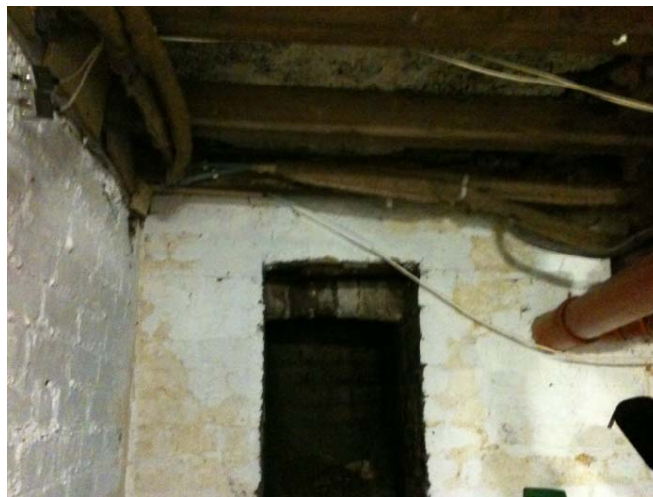
Figure 11: Existing cellar, opening of redundant coal chute
