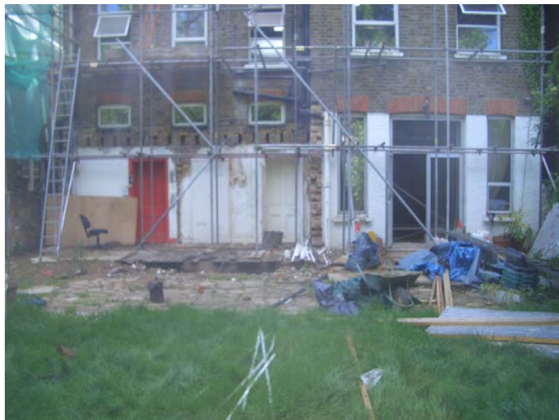
Figure 5: Partial view of rear garden looking towards rear of building
