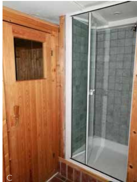
Photos A-C Photo A shows the staircase. Photo B shows a new pier column which supports a new beam. Photo C shows timber partition between the sauna and shower.
