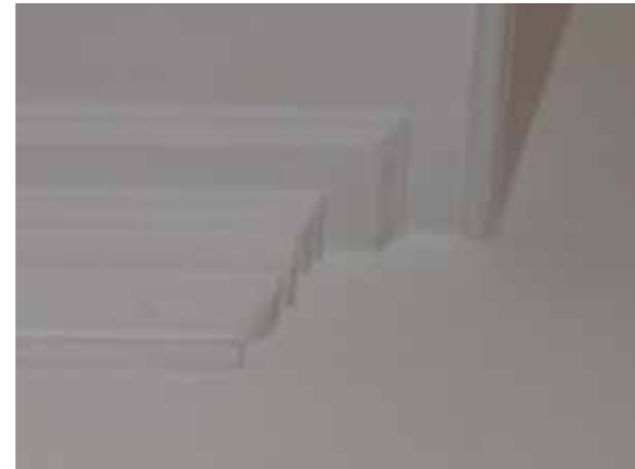
Moulded cornice detail abutting stair
