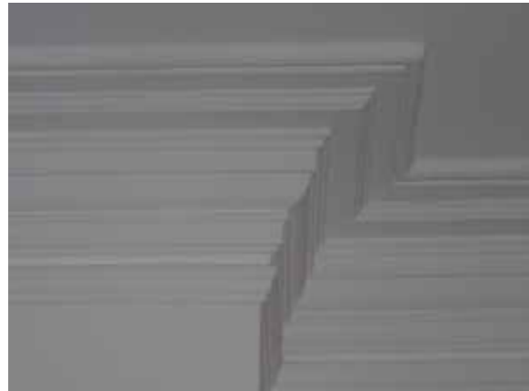
Moulded cornice detail to the ceilings
