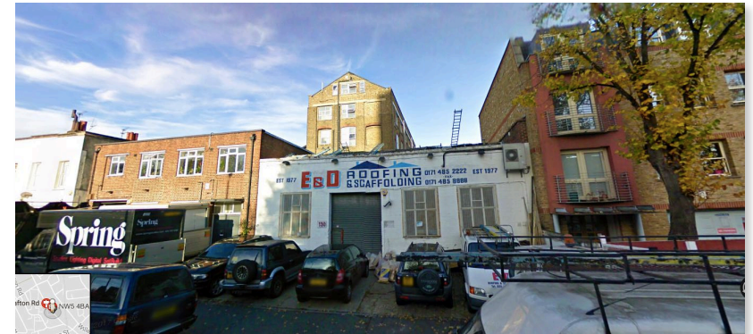
EXISTING SITE (photograph)
