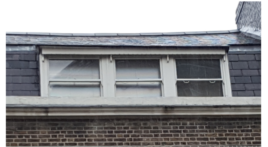
External Blind Box at 61 Doughty Street
