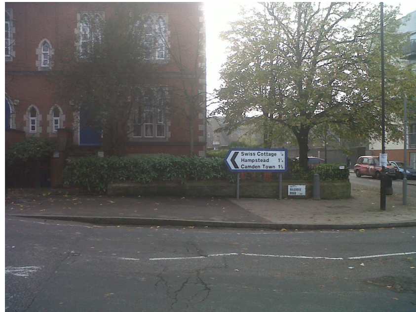
LOCATION WITHOUT POLE Dwarf wall and railings to 22-24 Hilgrove Road
