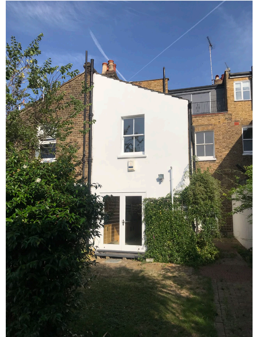
Rear of 5 Achilles Road
