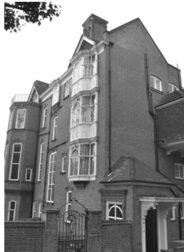
6 Ellerdale Road by Richard Norman Shaw
