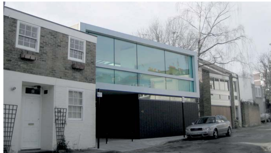
MSA Project Kingstown Street, London NW1 8JP
