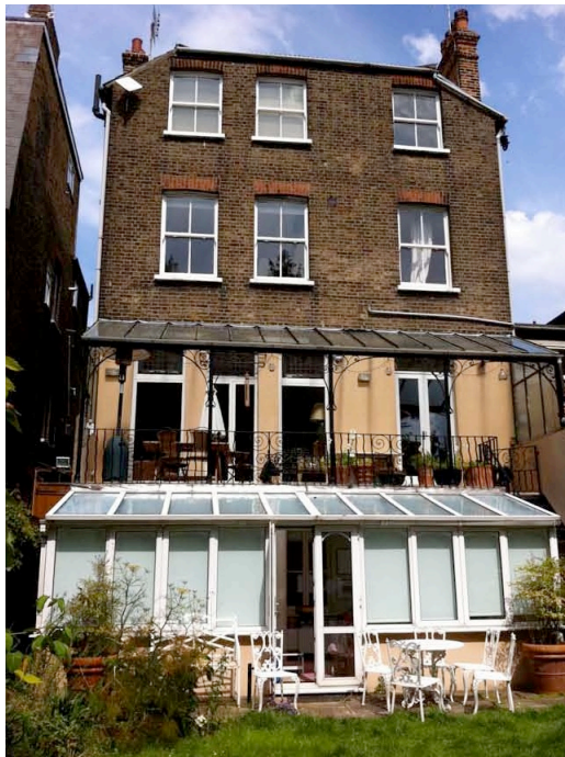
Rear elevation showing existing extension
