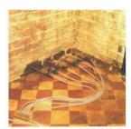
The wall area shall then be pressure injected using a specially formulated solution of Kenwood siliconate injection fluid, until the entire depth of the wall is fully impregnated.
