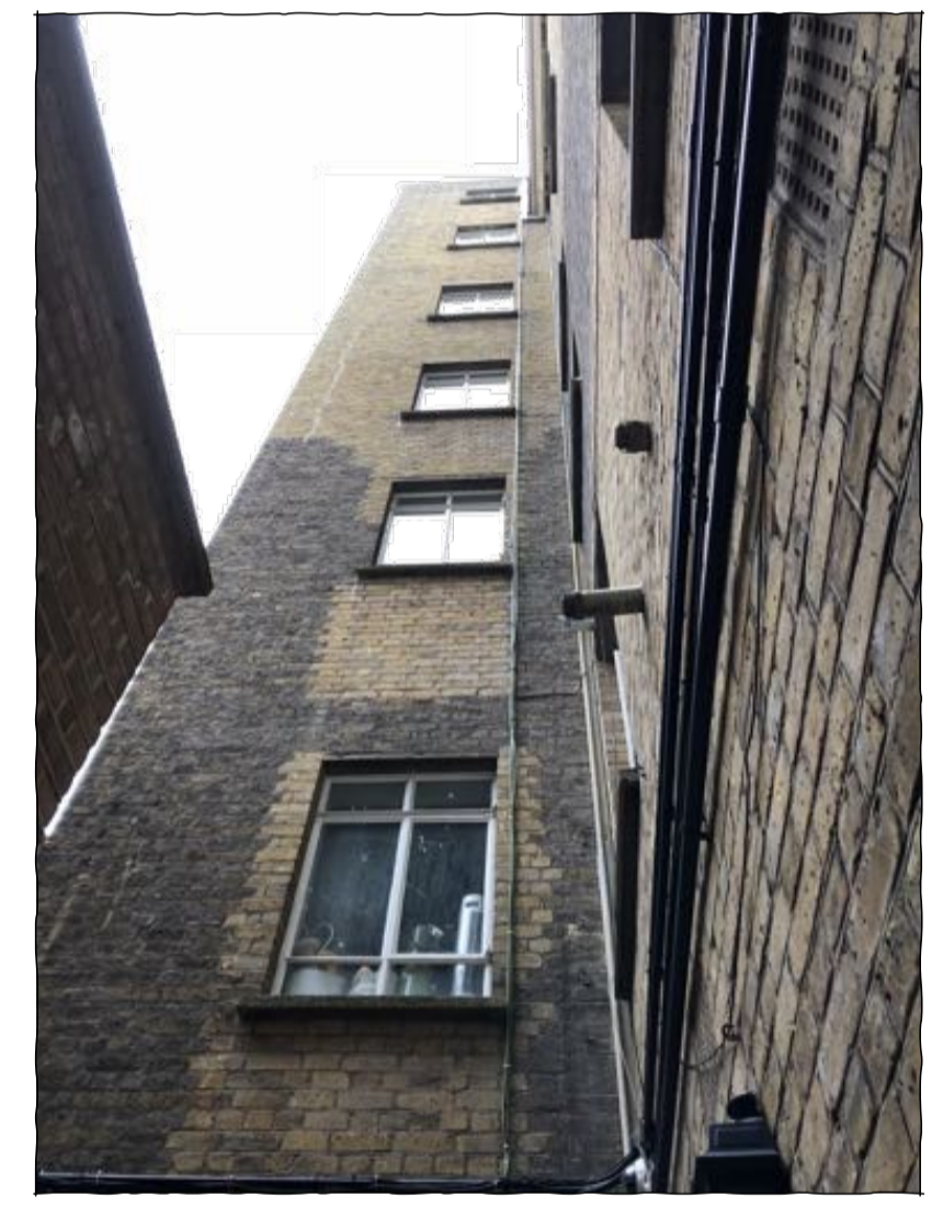
photograph A taken from basement ground level
