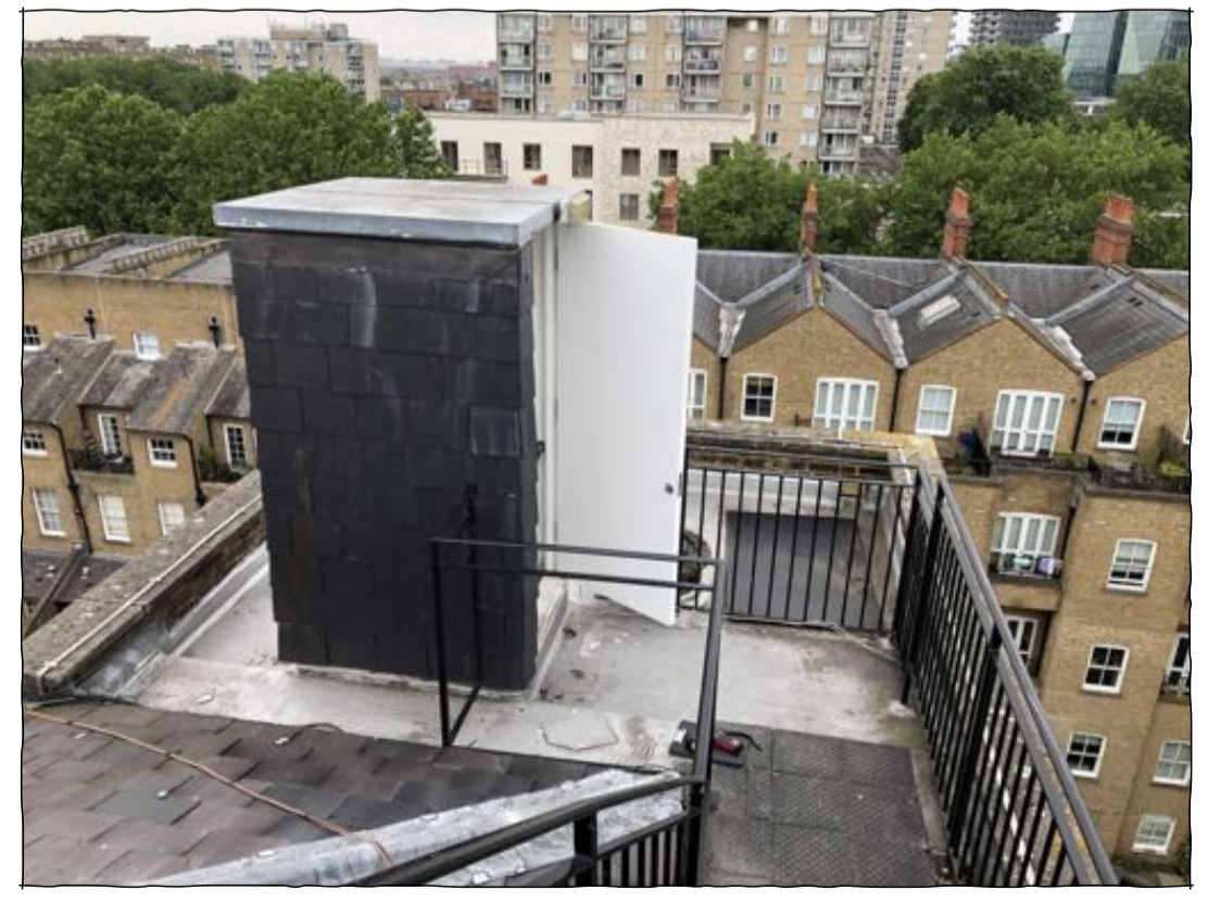
photograph B taken from lightwell bridge level
