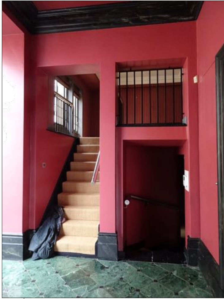
central separating partition removed opening increased in width and height. skirtings, architrave and cornice removed
