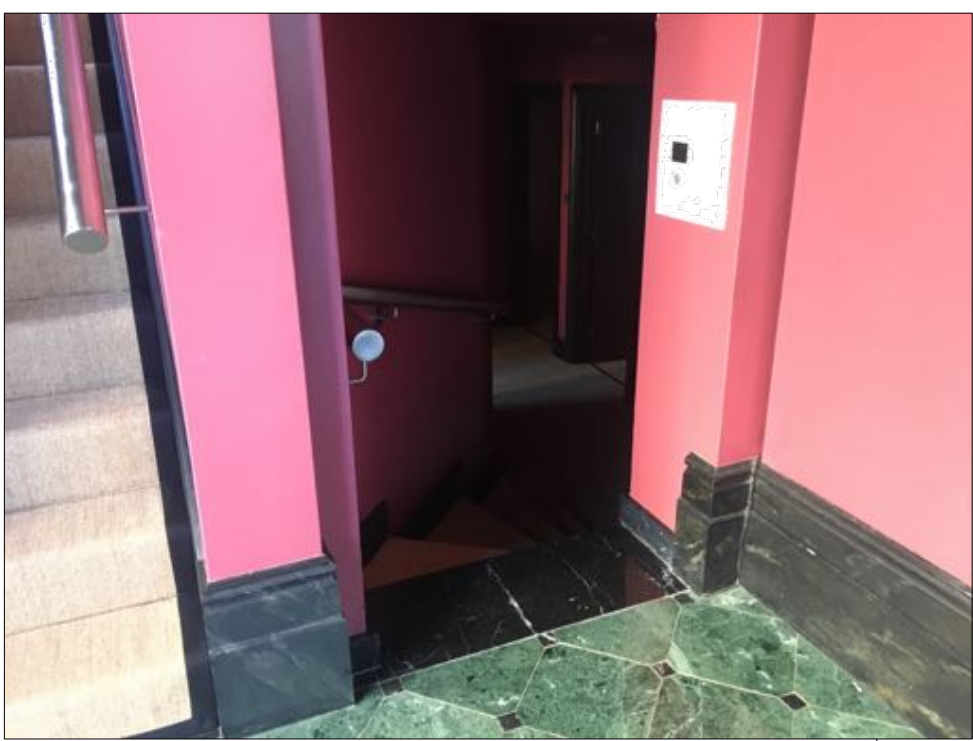
stair opening increased in width with dividing wall removed, stairs removed, skirtings and architraves removed
