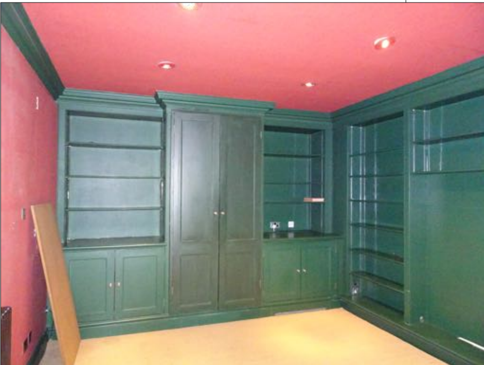
joinery, skirtings and corning removed
