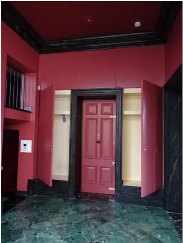
joinery around entrance door removed allowing increase in width for stair opening. flooring, cornice and architrave removed
