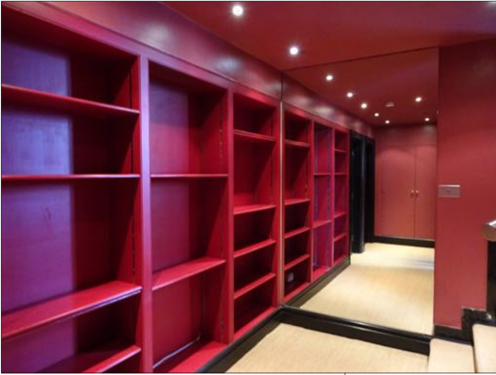
joinery, partitions, floor finishes and stairs removed
