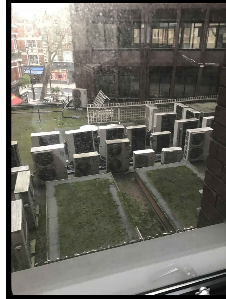
PHOTO VIEW 01. POST SCAFFOLD & MONOFLEX
