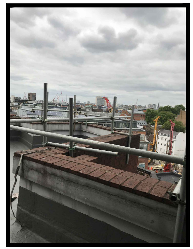
PHOTO VIEW 02. 8th FLOOR ROOF VIEW
