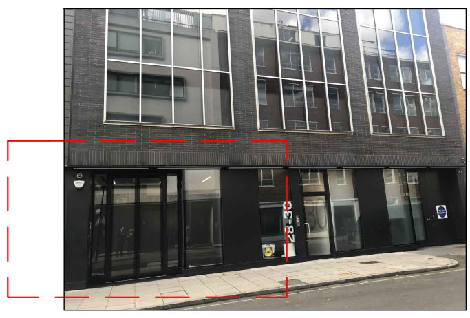
EXISTING FRONT ELEVATION PHOTO SCALE 1:50
