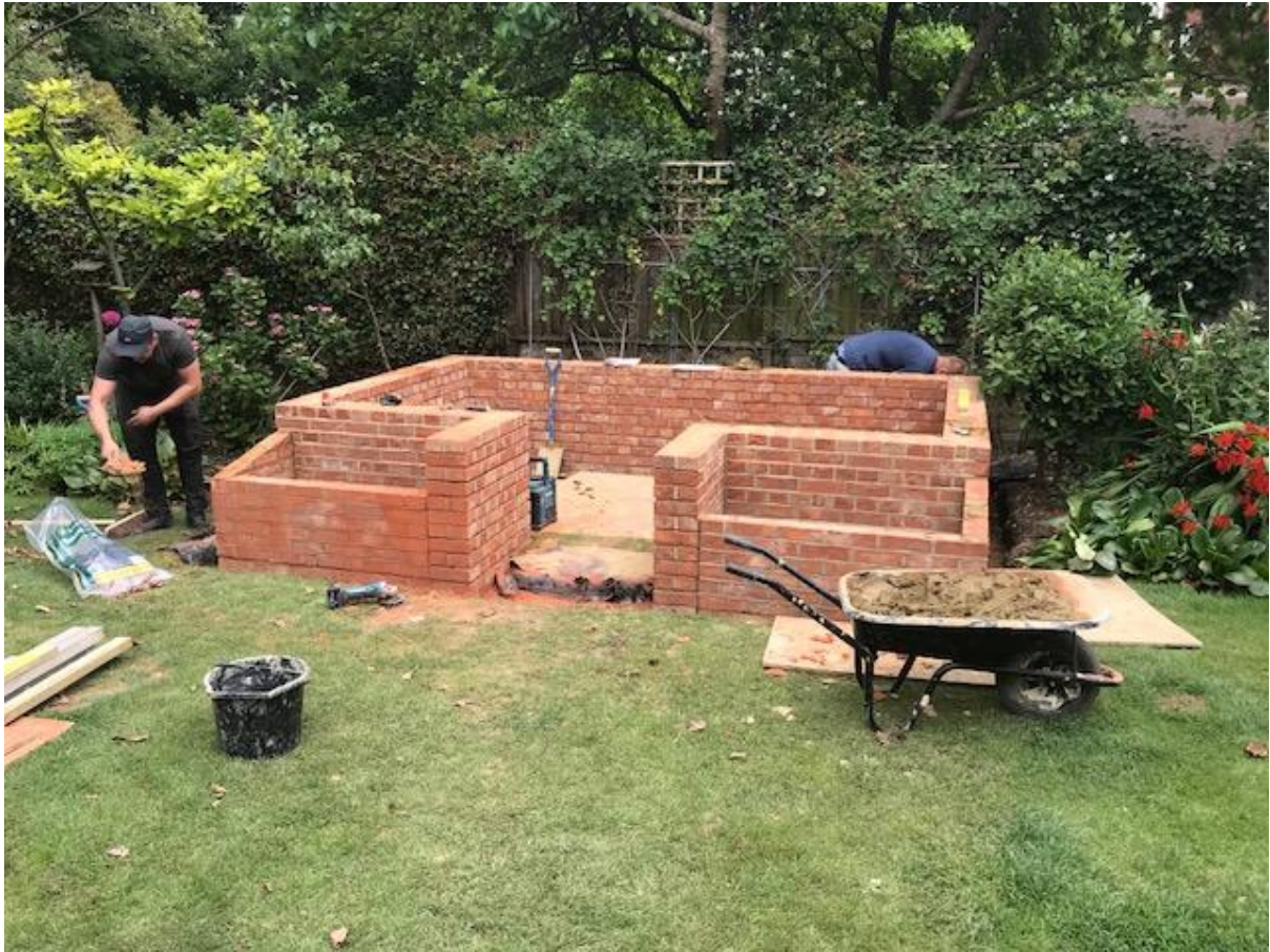
Trenches for wall were cut as narrow as possible to minimise disturbance. Also note condition of surrounding grass. Only hand tools used no machinery to dig.
