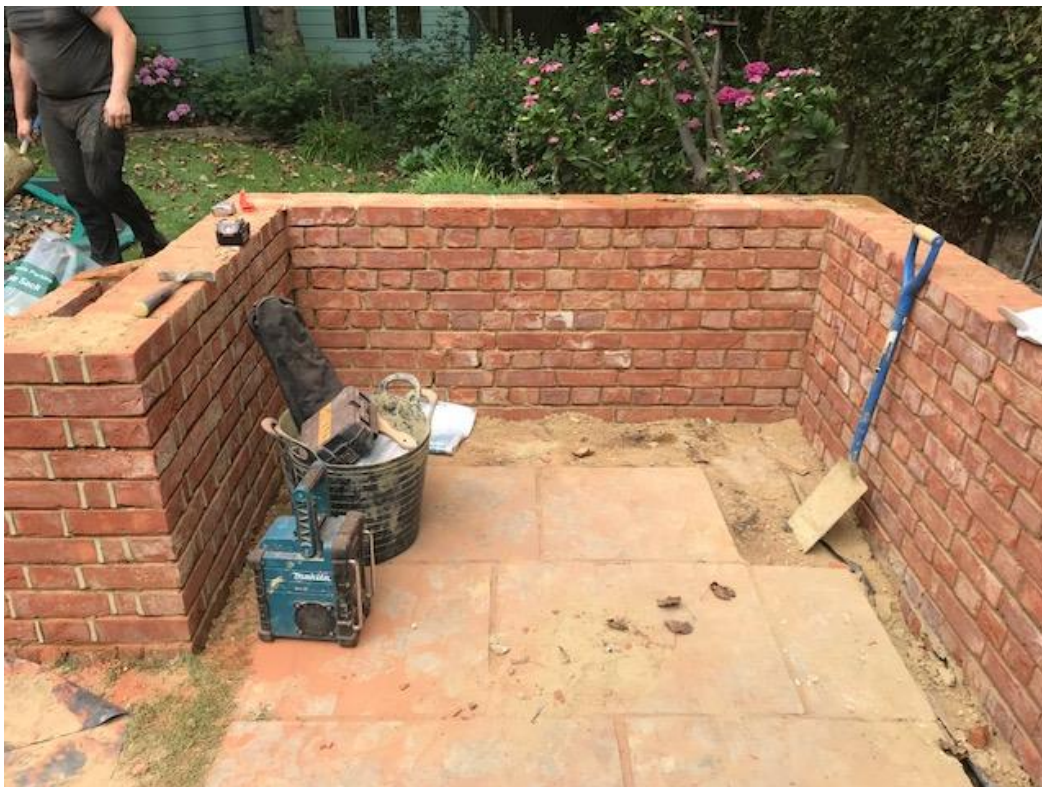
Internal view after wall built showing original paving minimally disturbed.
