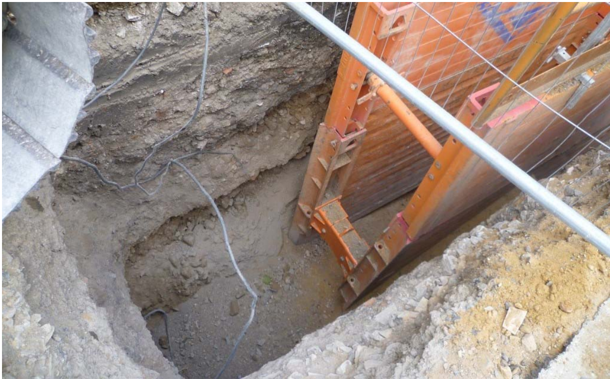
Photo 4 Deep drainage trench, looking north
