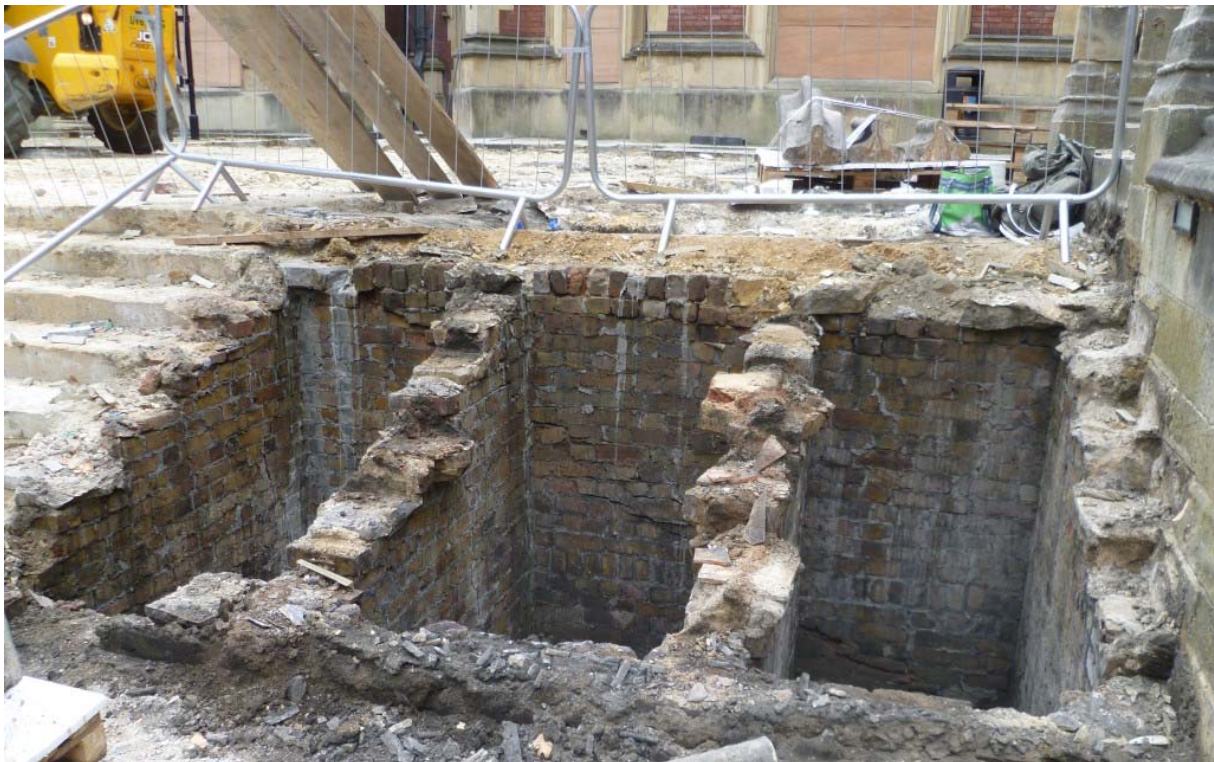
Photo 1 Steps with voids below northern three sections
