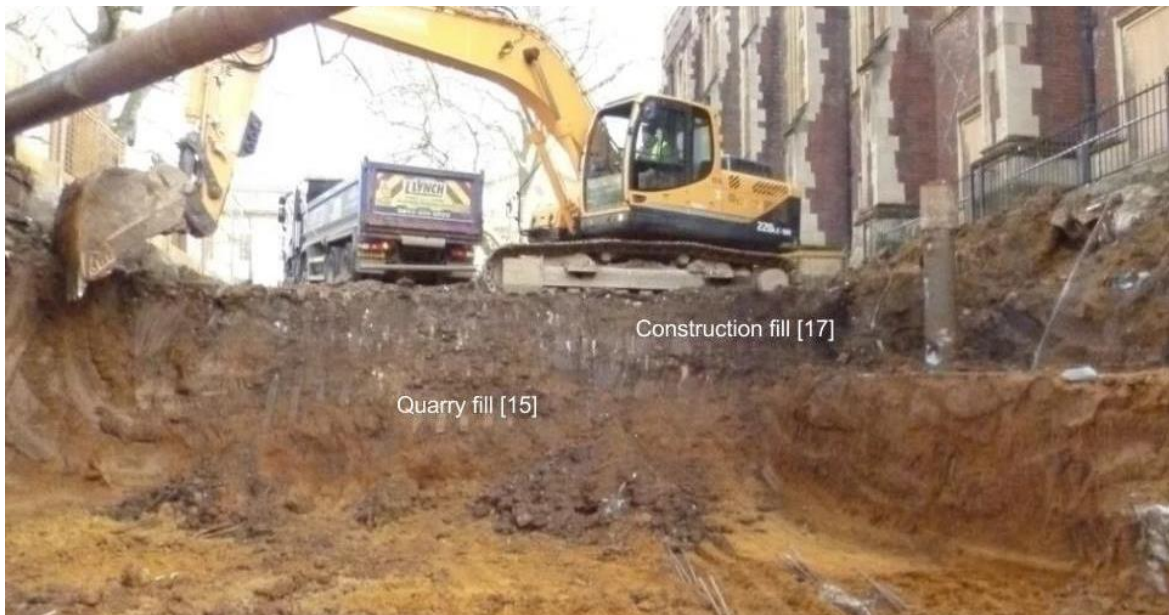
Photo 6 Excavating brickearth quarries beneath the former Under Treasurer's House
