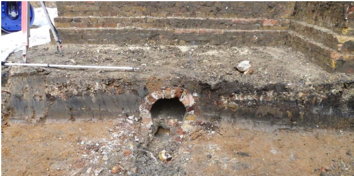
Photo 7 19th-century brick drain built at the time of construction of the Great Hall and possibly at the base of a large construction cut indicated by the change in the colour of deposits
