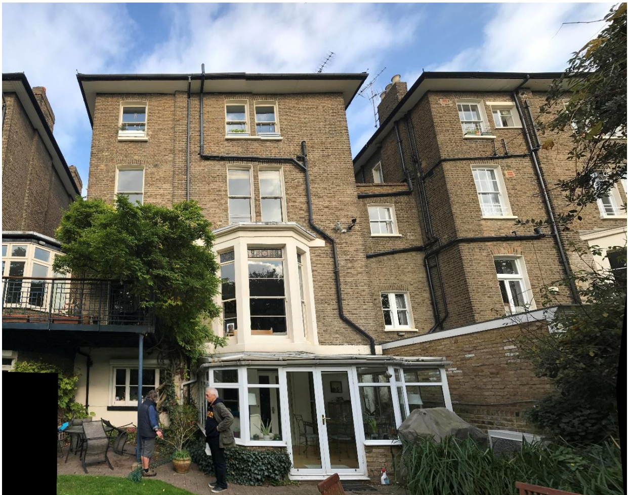
Rear elevation of 141 King Henry's Road
