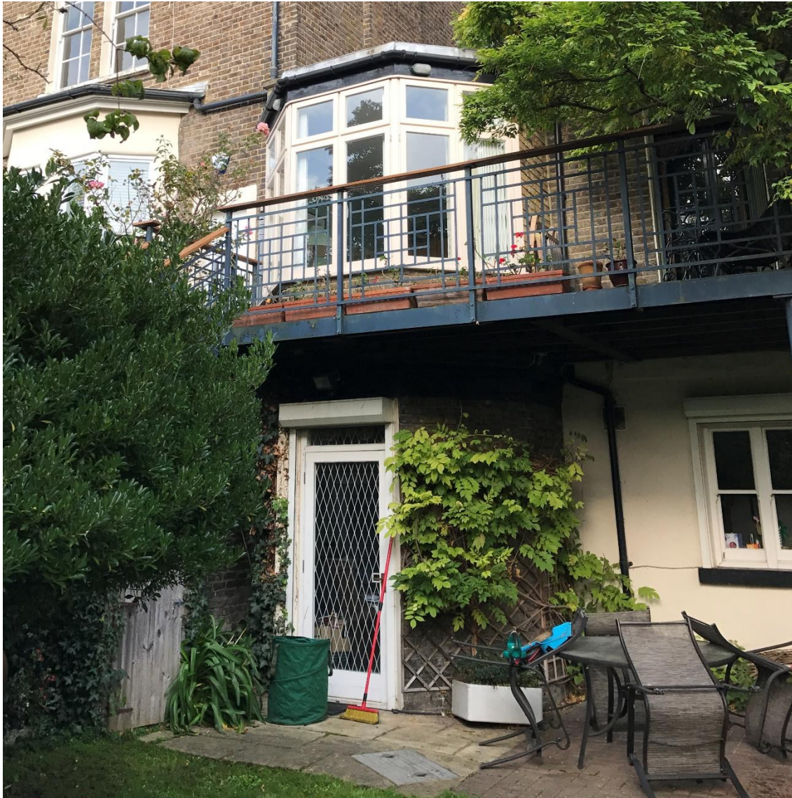
Rear elevation of ground floor bay at 141 King Henry's Road
