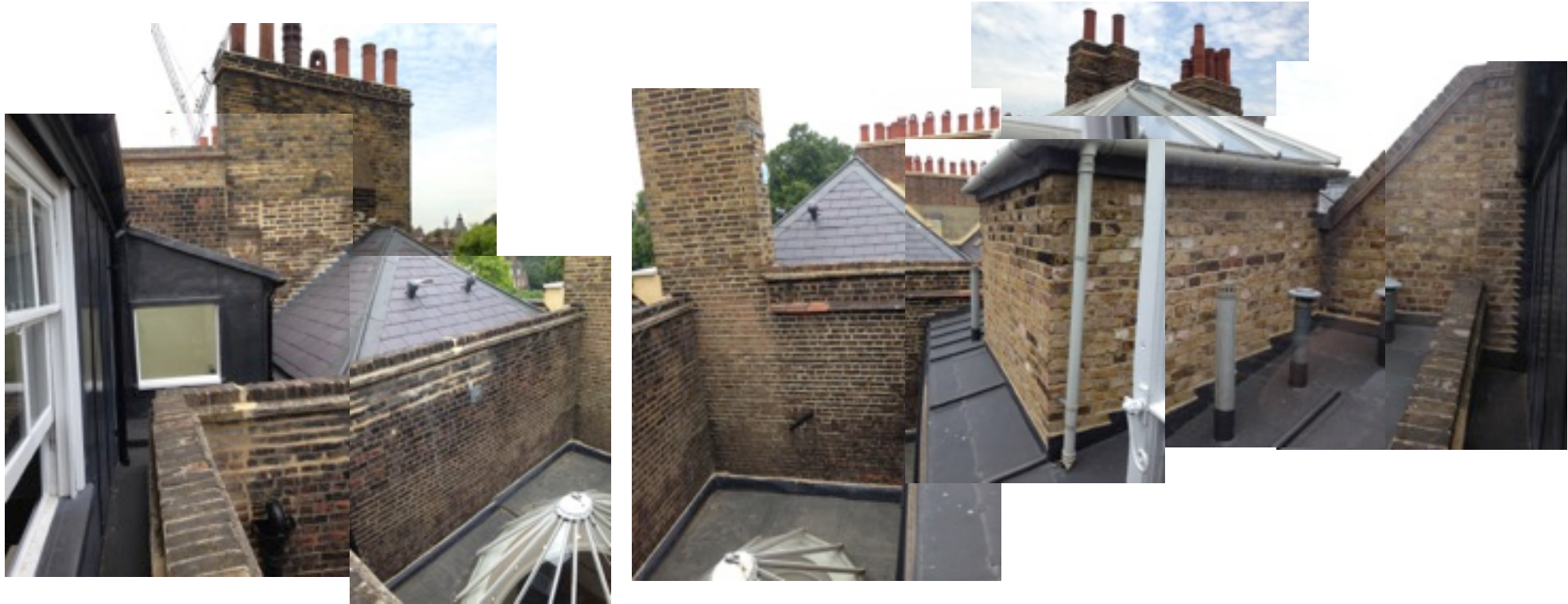
LIGHT WELL AT THIRD FLOOR
