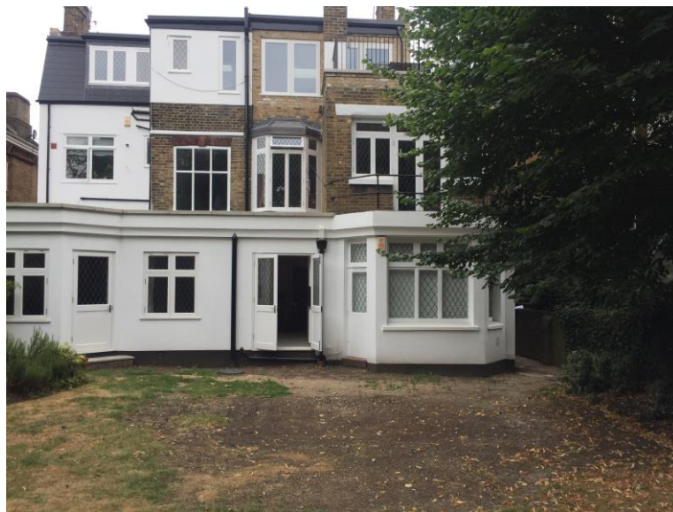
Rear view of 103 Priory Road
