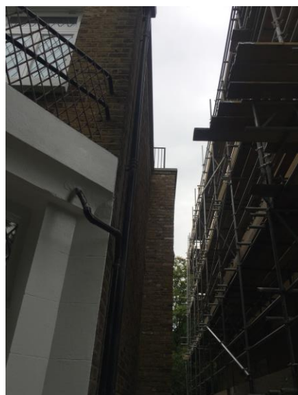
View side extension looking east
