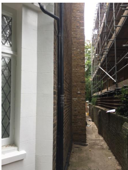
View of side extension looking east
