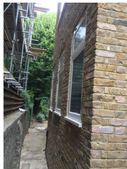
View of side extension looking west
