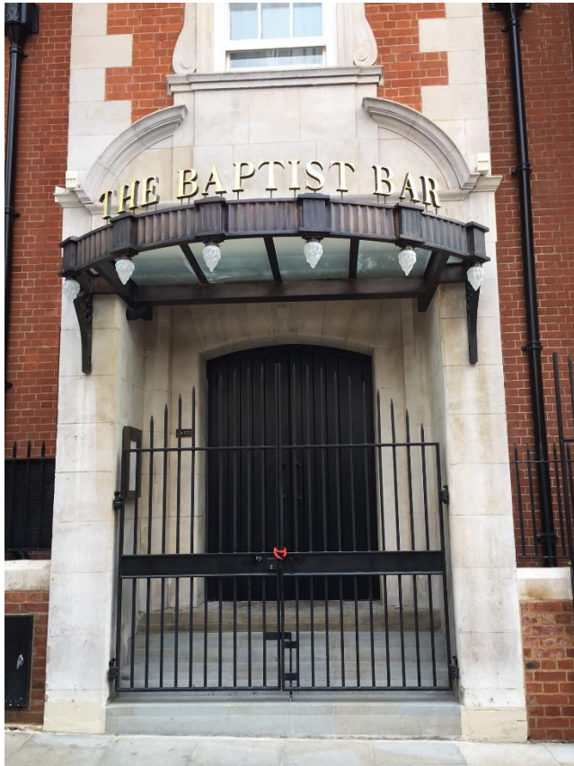
Existing Glazed Canopy above Hotel Restaurant Entrance, Catton Street.
