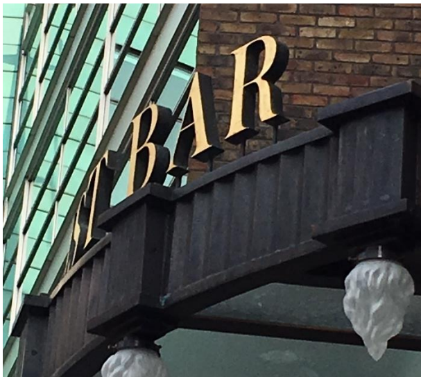
Detail of lettering format and finish – individual letters with 30mm depth. Front face finished in Antique Gold, depth/return sides of lettering in Antique Bronze to match canopy fascia.
