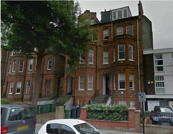
Fig.1 – View of primary elevation from Fellows Road
