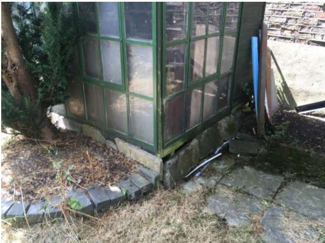
Photograph 4: Glass Fronted Shed at 63 Hillfield Road, London
