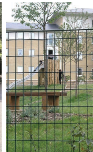
STEEL GRATING FENCE
