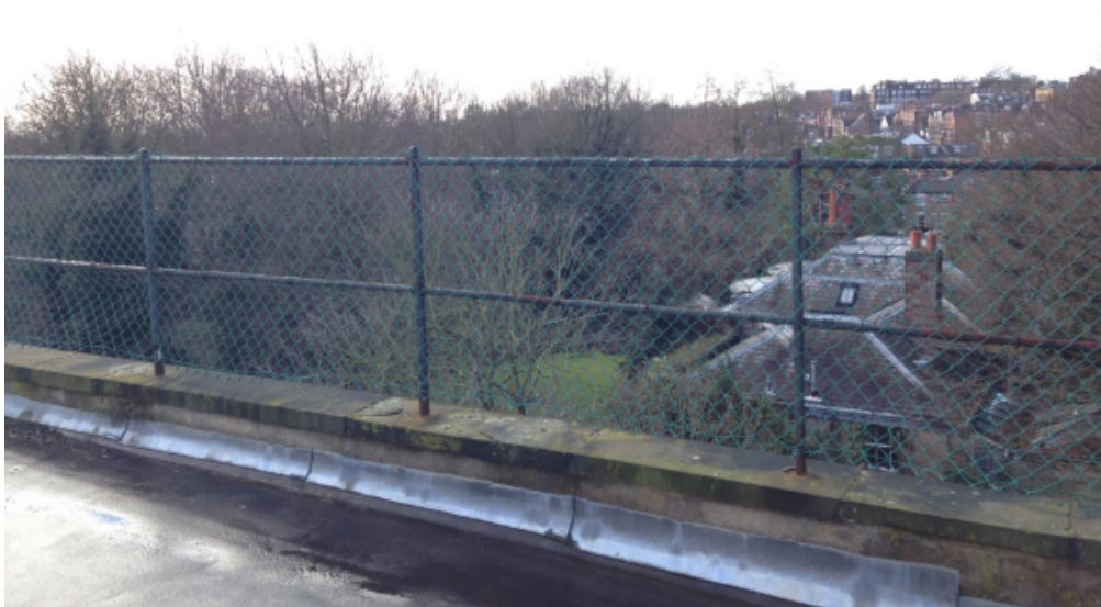
8. Roof terrace with existing railings
