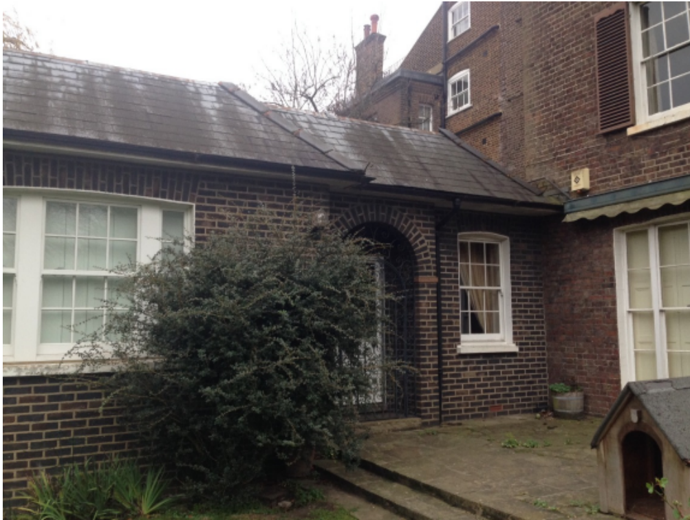
7. Existing rear extension
