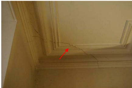
Communal Stairs – Diagonal Crack below window
