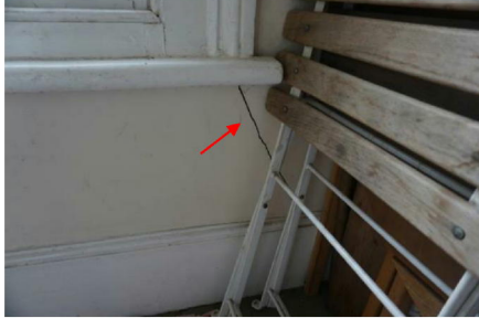
Communal Stairs – Diagonal Crack below window
