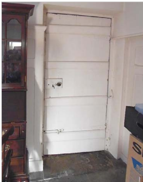
Figure 3.9: Original door within front room (February 2016)
