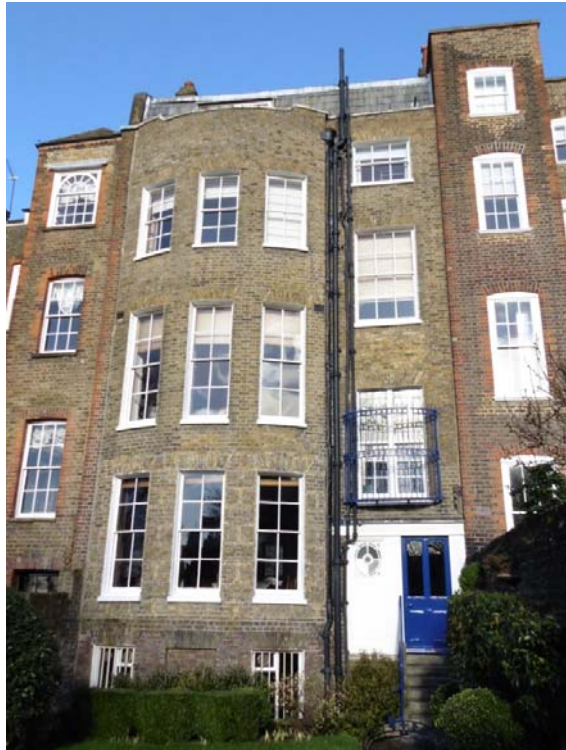
Figure 3.31: Rear elevation (February 2016)
