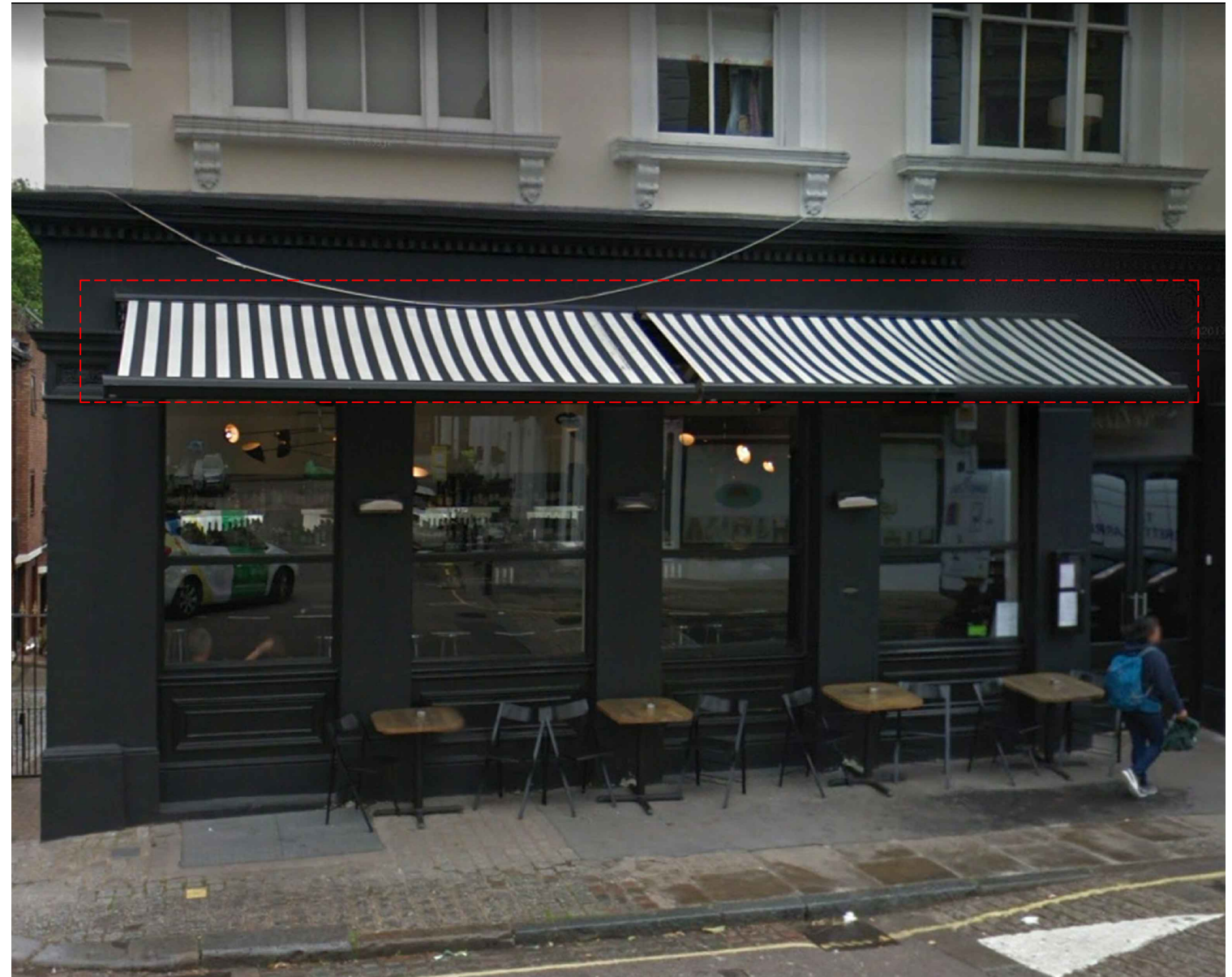
Canopies to be removed and background made good
