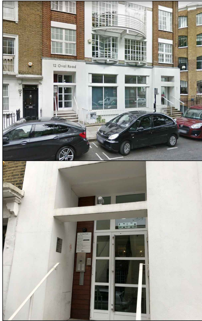
Existing Images of Entrance Door
