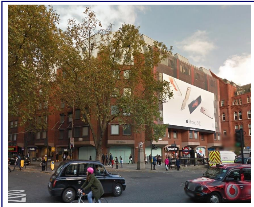
General view of the site (facing northeast).
