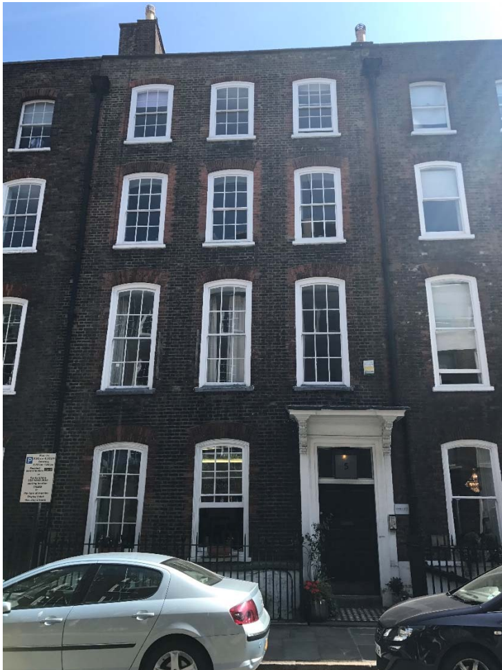
Fig 1 Street View: 5 Great James Street
