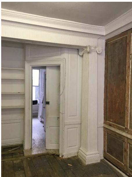
Fig 7 Existing Non-original Lobby to RM.0.2
