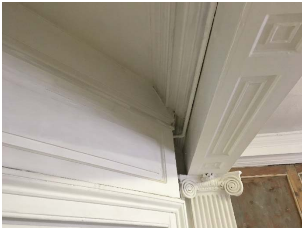
Fig 9 Lobby partitions interfacing with historic cornice above
