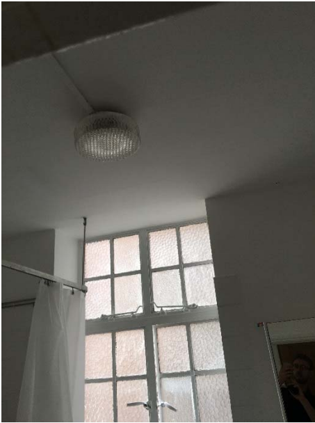
Fig 13 Non-original metal frame window W.1.5 and dropped ceiling in Bathroom RM.1.7
