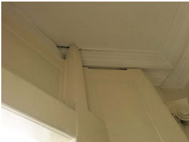
Fig 10 Storage cupboard interfacing with historic cornice above
