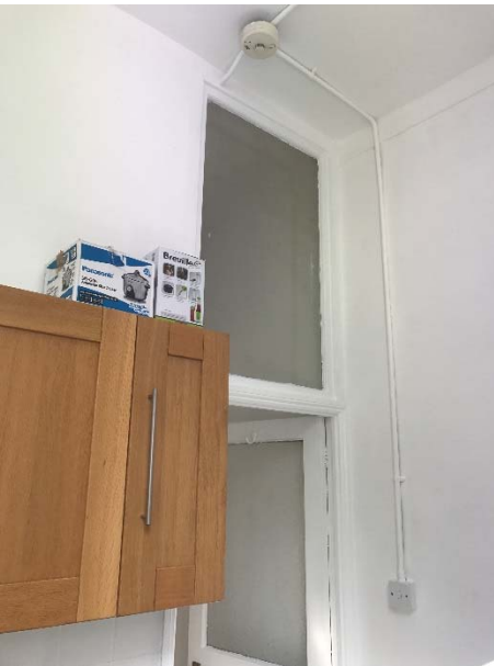
Fig 17 Existing non original wall partitions between kitchen and hallway
