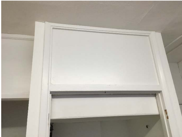
Fig 5 Unused water tank above kitchenette
