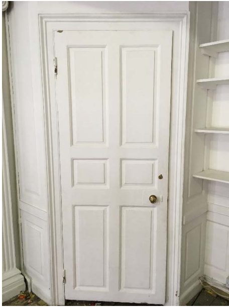
Fig 8 Existing Non-original storage cupboard in RM.0.2
